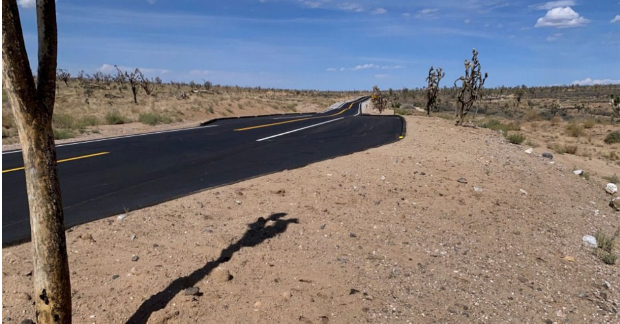
FIGURE 3. EXAMPLE OF A SIMILAR PULLOUT AREA RECENTLY COMPLETED ON CIMA ROAD IN THE PRESERVE
