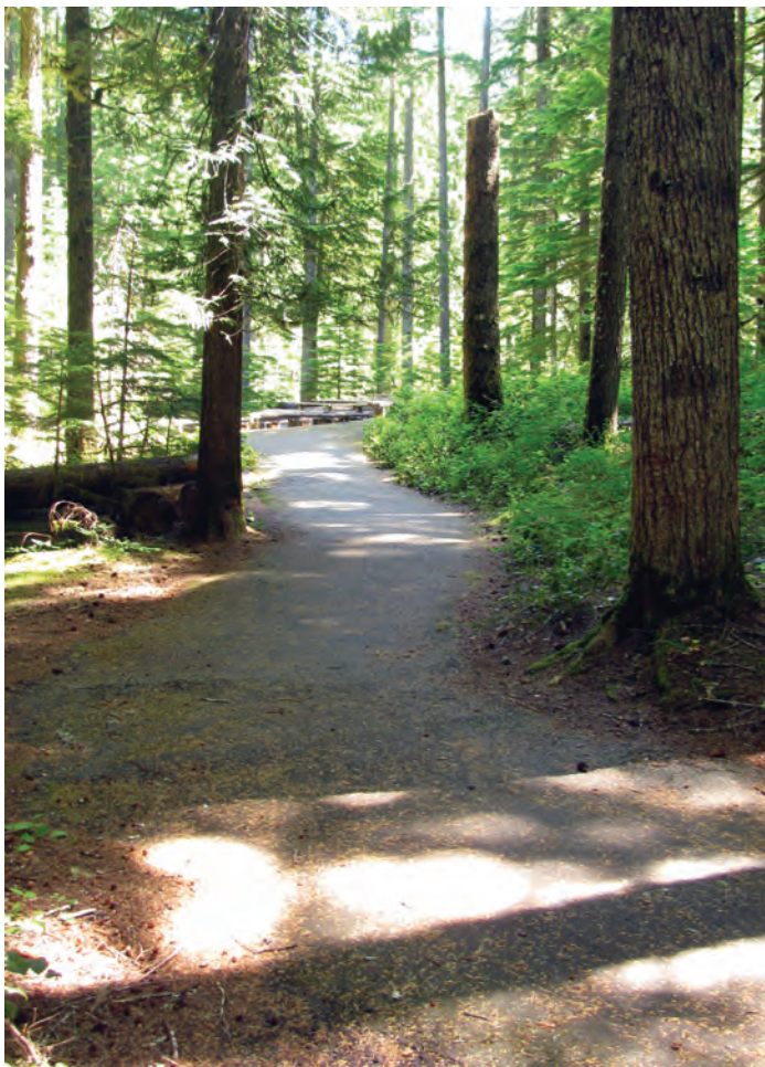
Figure 55. Asphalt path leading to amphitheater, 2017. Source: NPS.
