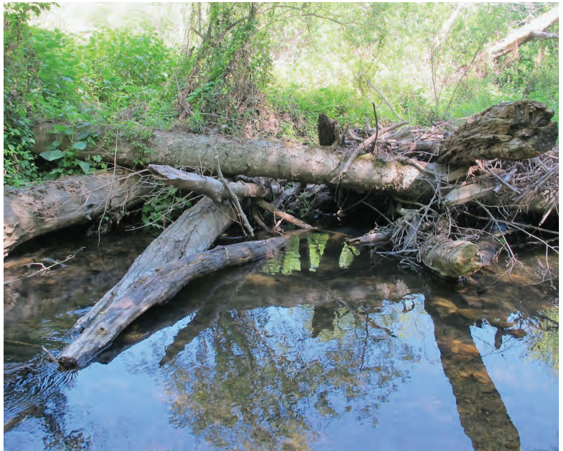
Figure 39. Large woody debris in a "jackstraw" pattern, used to protect a stream bank and improve habitat. Source: fishbio.com.
