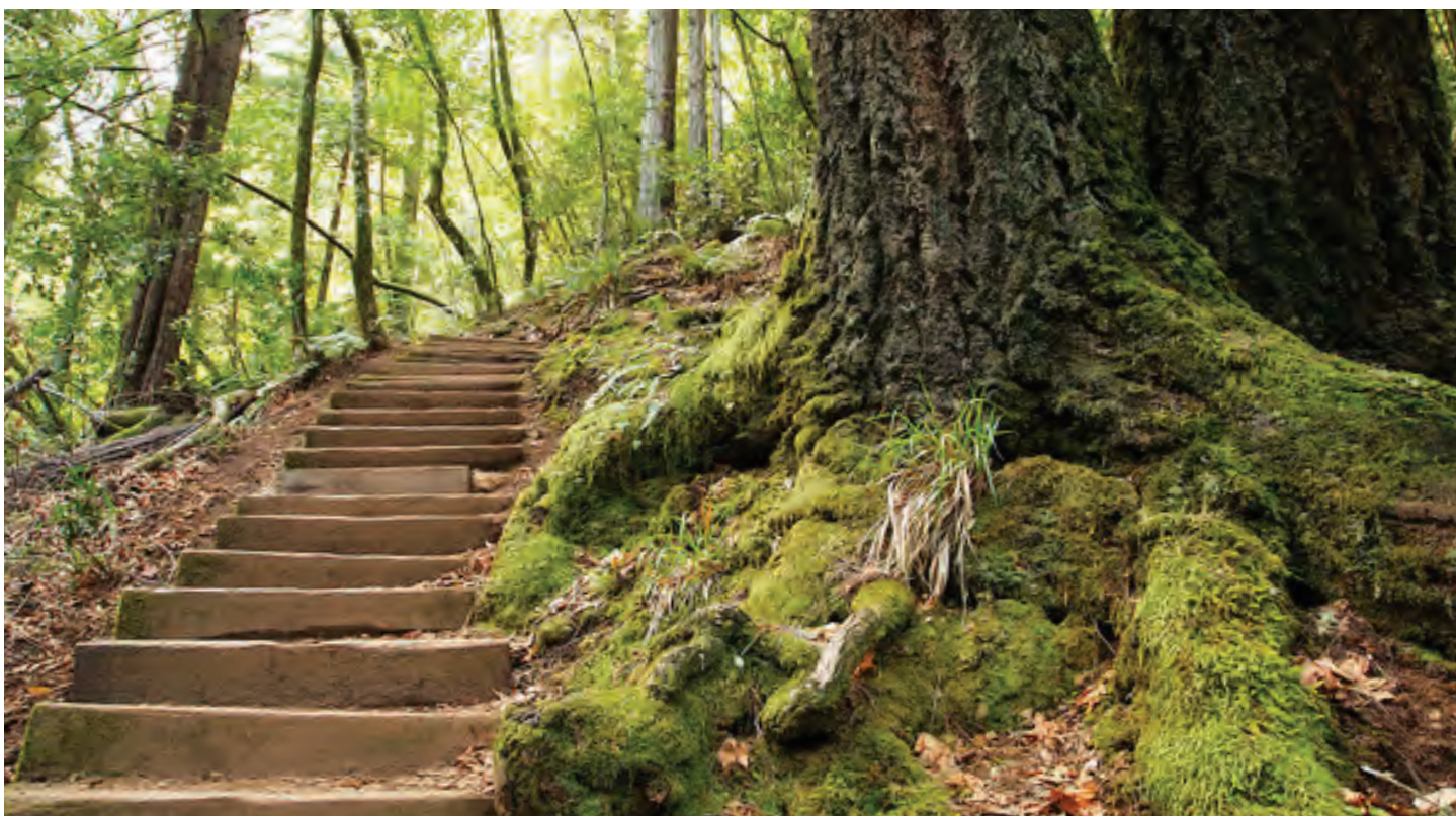
Figure 61. Example of box steps created from milled lumber, Cataract Falls Trail. Source: eastbaytrails.com.
