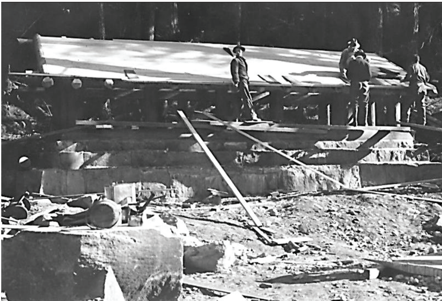
Figure 10. Construction of a comfort station at Ohanapecosh, 1934. Source: NPS 2016.
