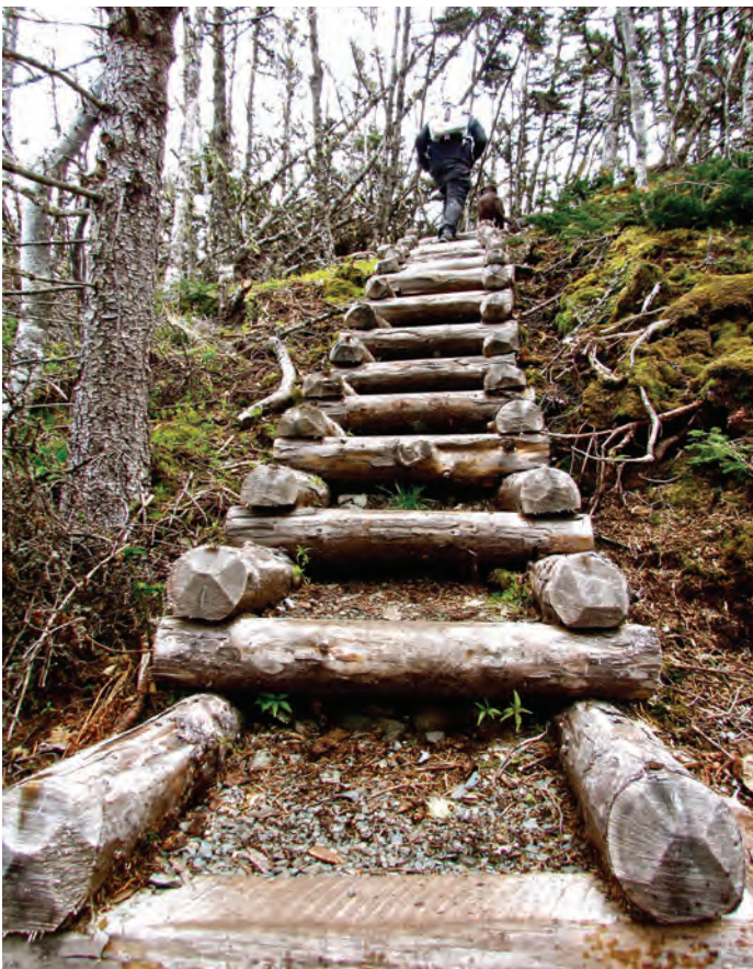
Figure 64. Example of steps built from logs, Skerwink Trail, Newfoundland. Note the scoring on the first tread to improve traction. Source: adventuresinnewfoundland.wordpress.com.
