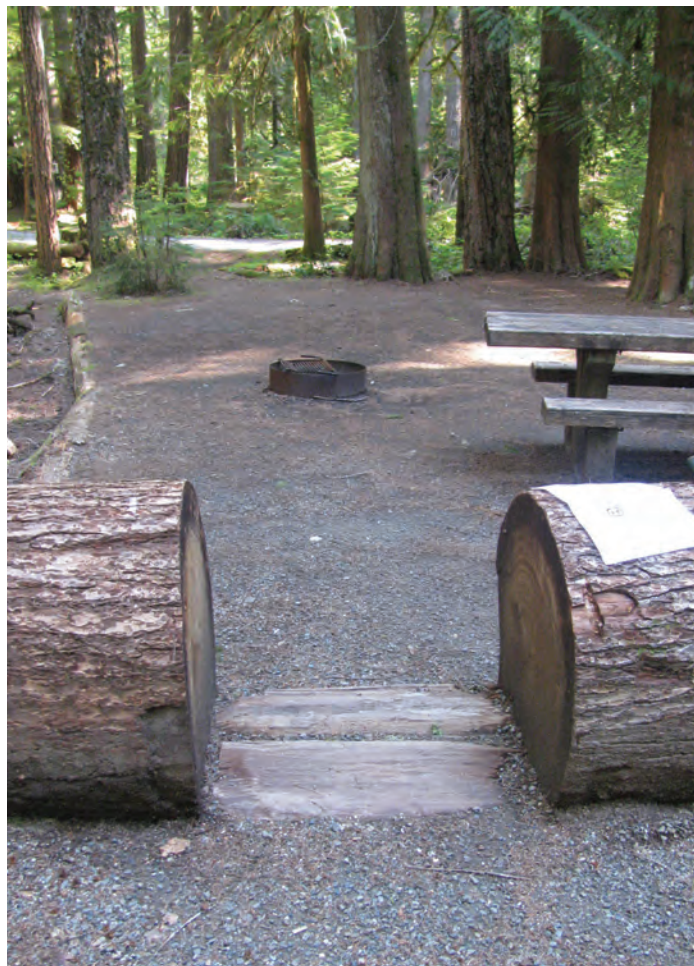
Figure 56. Newly resurfaced campsite, 2017; forest duff begins to accumulate in the compacted gravel. Source: NPS.
