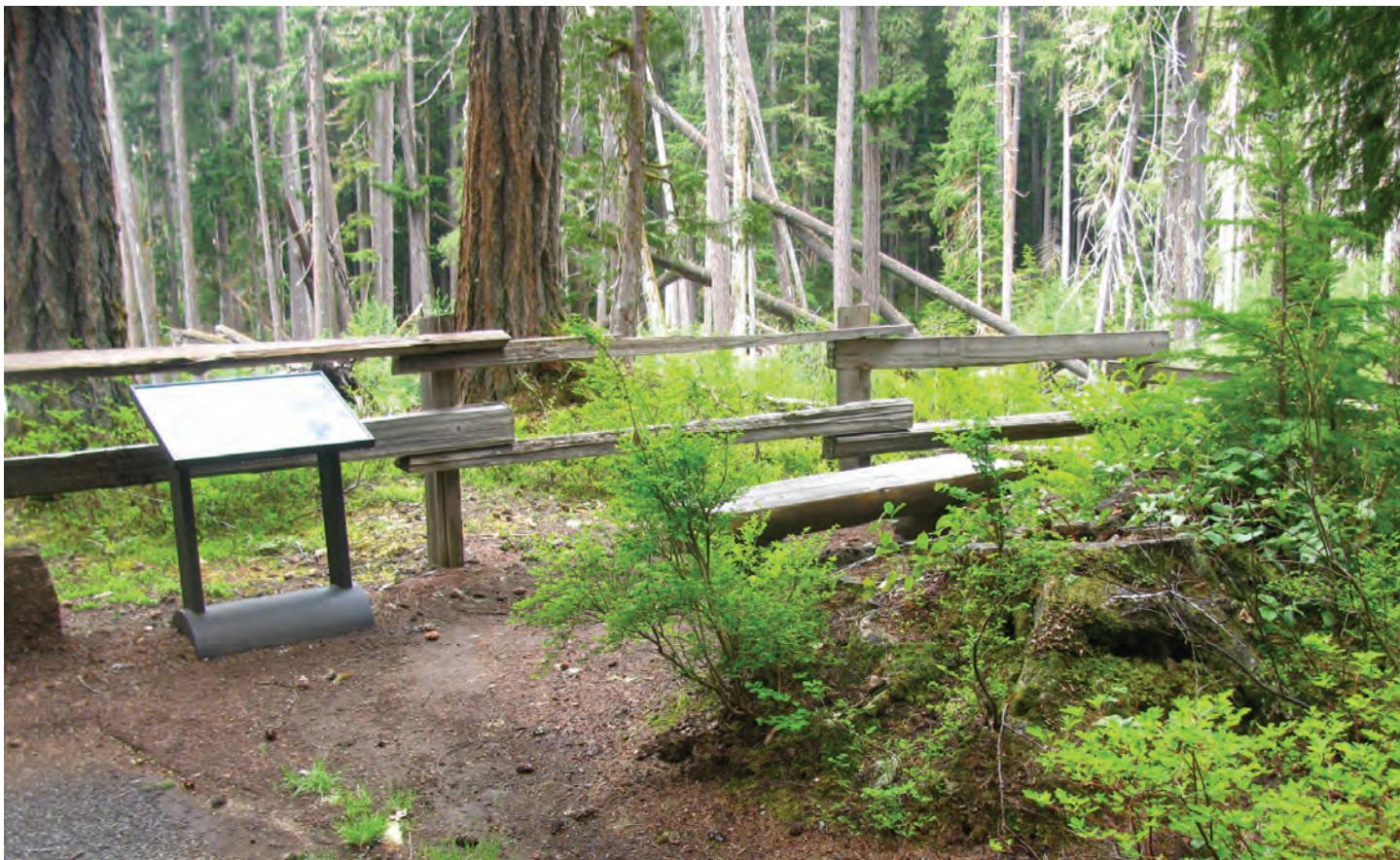
Figure 60. Split-rail fencing is an appropriate edging choice if a higher barrier is desired. Source: NPS.
