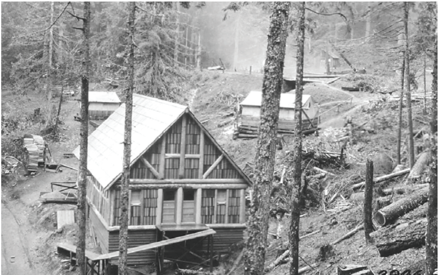
Figure 5. The Ohanapeosh Hot Springs Resort Bath House Under Construction, 1927. Source: NPS 2016.
