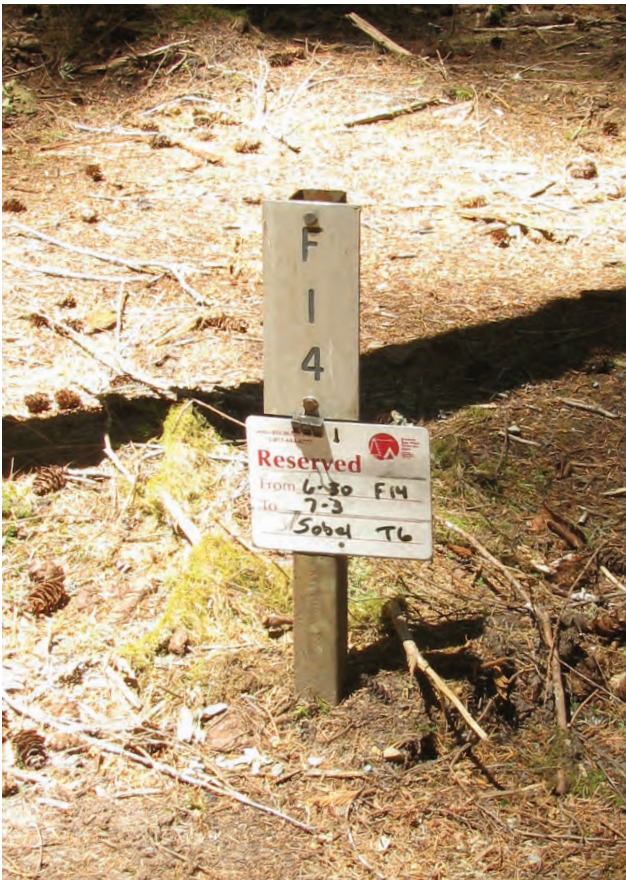
Figure 83. Existing campsite identification signs with sharp metal corners, 2017. Source: NPS.
