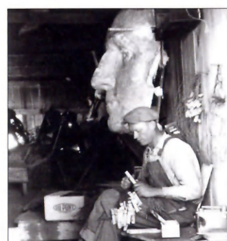
Art Johnson prepares dynamite for blasting granite.
