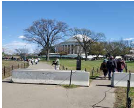
Photo 2. Temporary Jersey barriers at Jefferson Memorial (photo by Land Collective)
