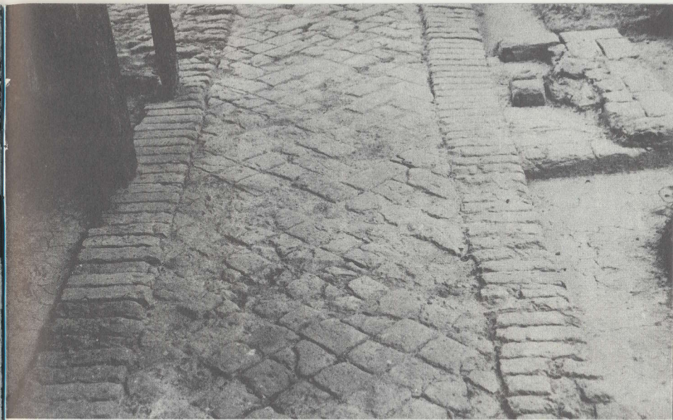
Brick, fired at the nearby kiln, were used in walks, chimneys, and steps.
