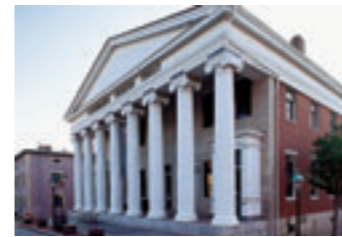
Double Bank Building
