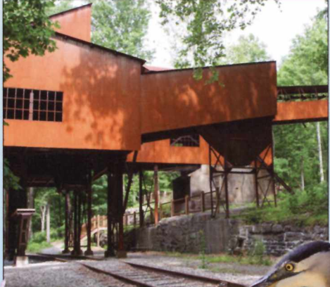
Abandoned mining structure in Nuttallburg NPS / LOUISE McLAUGHLIN
