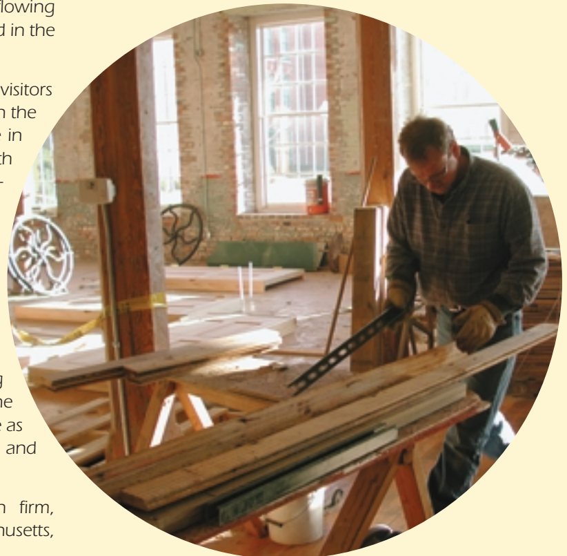
Installing Gift Shop floor.
