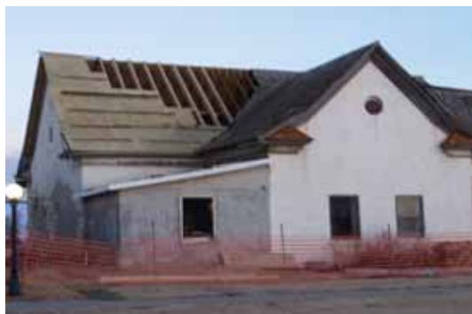
Rafters are strengthened and the roofing on the north-west side is underway, 2005.
