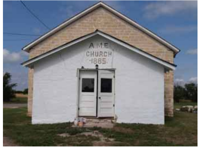
The A.M. E. Church - After
