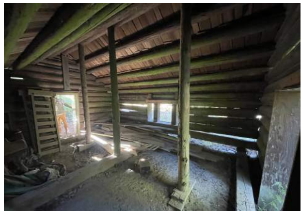
Image 37: Sleepers extend the width of the cabin.
