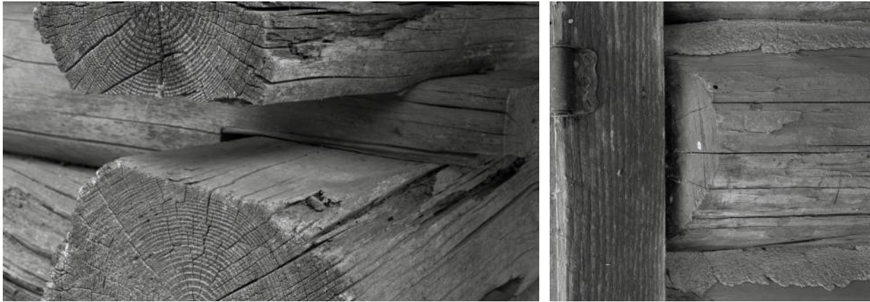
Image 50: Historic American Building Survey, log details, 2017
