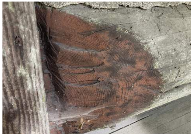
Image 42: Tooling detail at door surround on south elevation.
