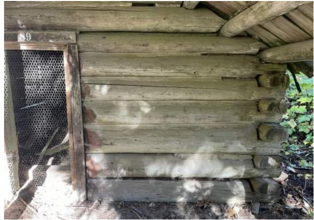
Image 29: The east portion of the south wall.
