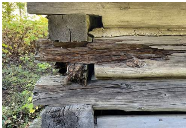
Image 34: The northwest exterior corner.
