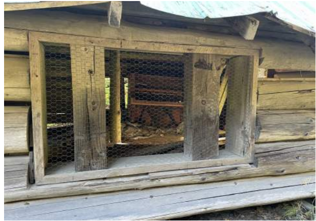
Image 38: The west elevation window opening.
