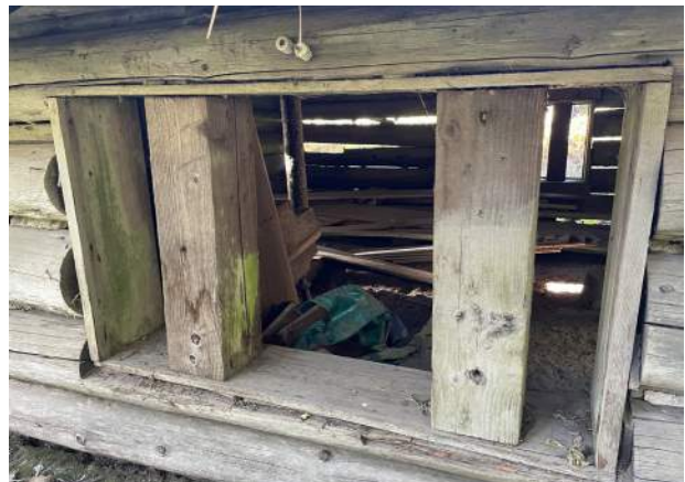
Image 39: East elevation window opening.
