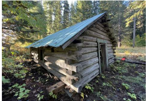
Image 26: Log walls connect with square notches.
