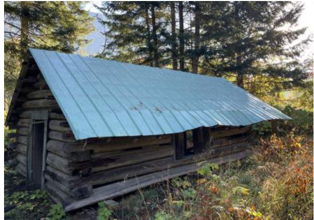
Image 19: A metal roof covers the original shake roof.
