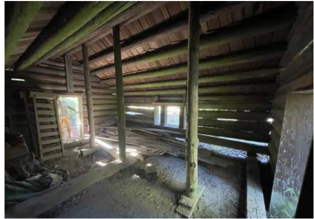
Image 45: The cabin interior is not finished.
