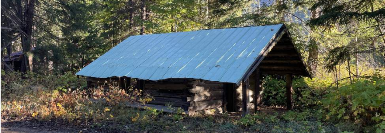
Image 10: The west and south elevations of the Courtney Cabin, facing north-northeast.
