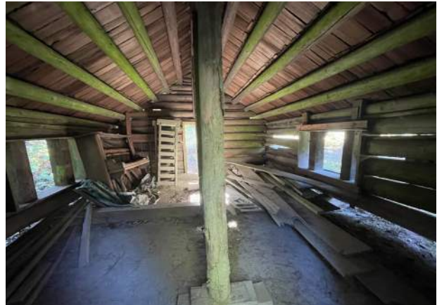
Image 11: Unfinished interior with dirt floor.
