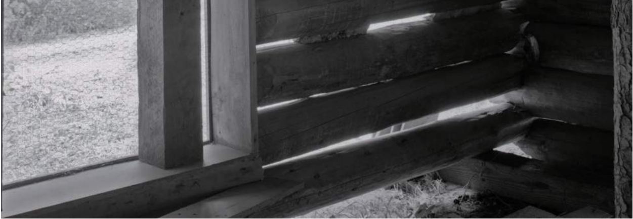
Image 48: Historic American Building Survey interior detail image, 2017
