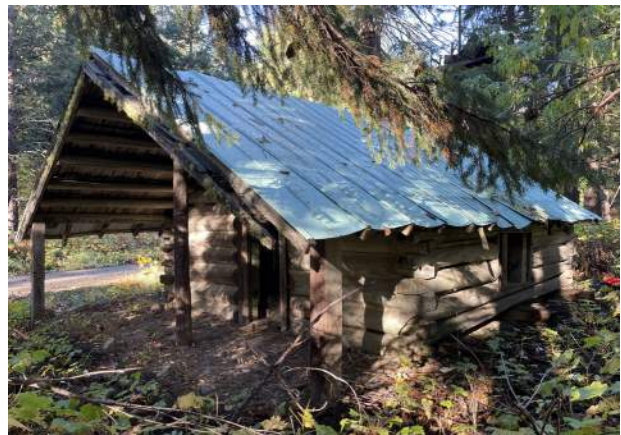
Image 12: Temporary shoring supports the porch roof and ridgepole.
