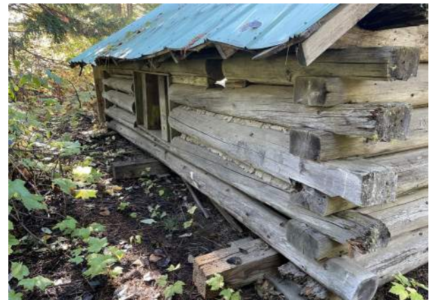
Image 27: East and west walls kept above grade with sleepers.
