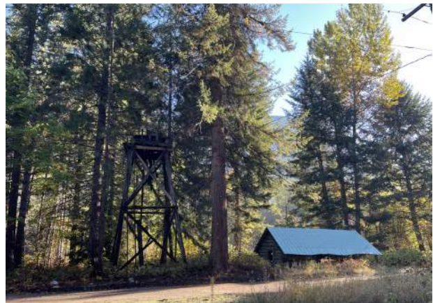
Image 18: A wood water tower remnant is north of the cabin.
