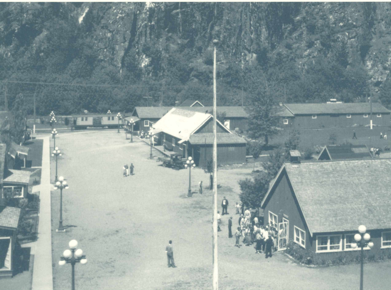
Looking south down Newhalem's Main Street, ornamental light standards with 5-globe clusters (SCL-L-122).
