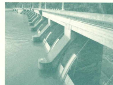
Detail of the tainter type spill gates, from the north end of Diablo Dam (WA-24-F-9).
