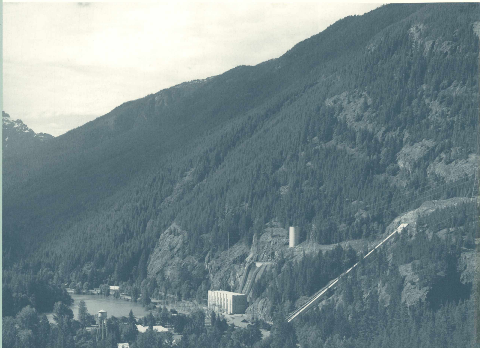
View of the community of Diablo from Highway 20. Visible features from left to right are the water tower, switchyard, Diablo Powerhouse, and the incline railway (WA-24-D-1).
