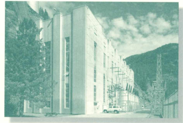
Diablo Powerhouse, dedicated in 1937. Aluminum-clad northern elevation designed as a temporary wall for possible future expansion (WA-24-D-2).
