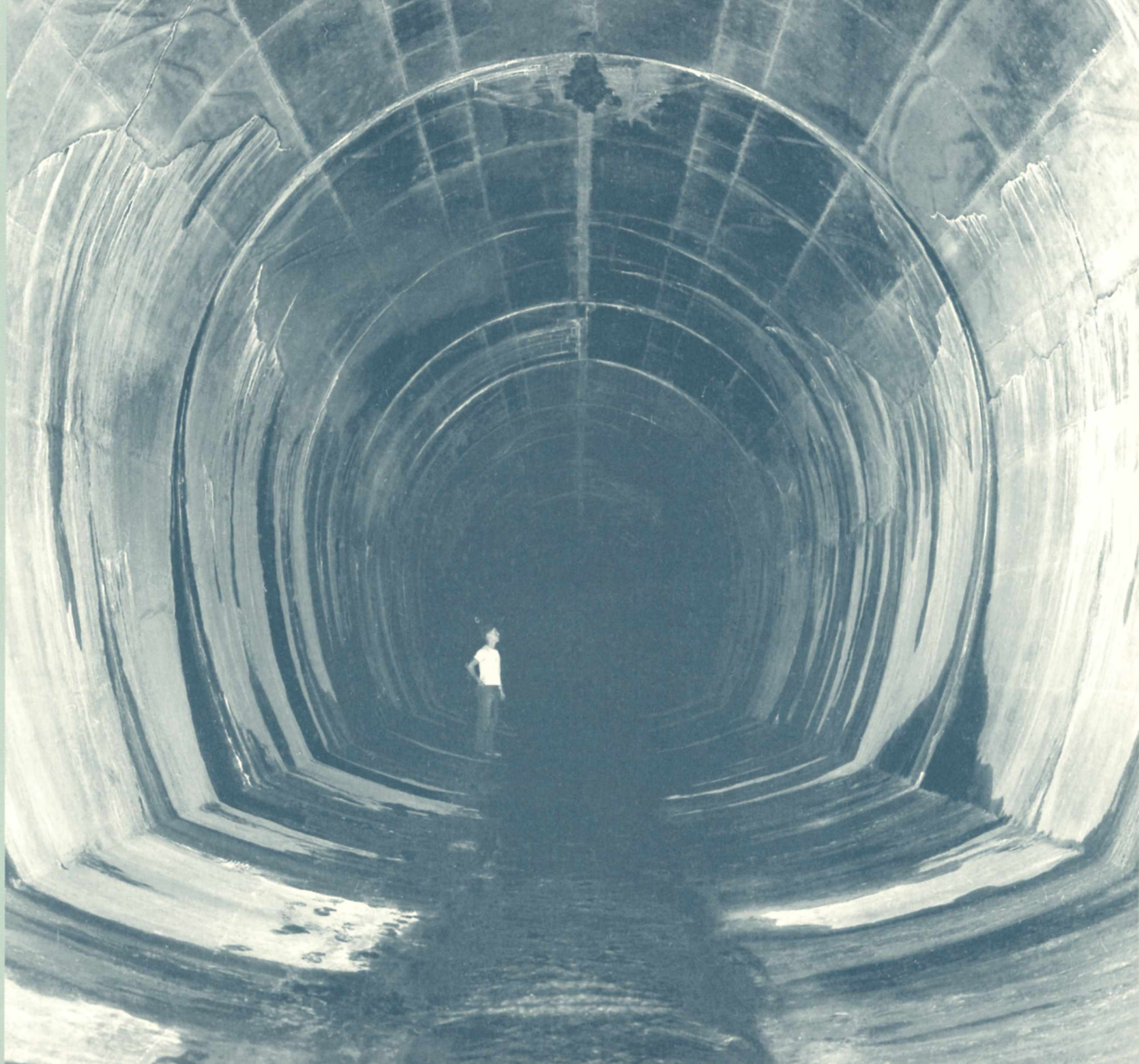
Interior of power tunnel during construction of Diablo Powerhouse, July, 1936 (SCL-LD-566).
