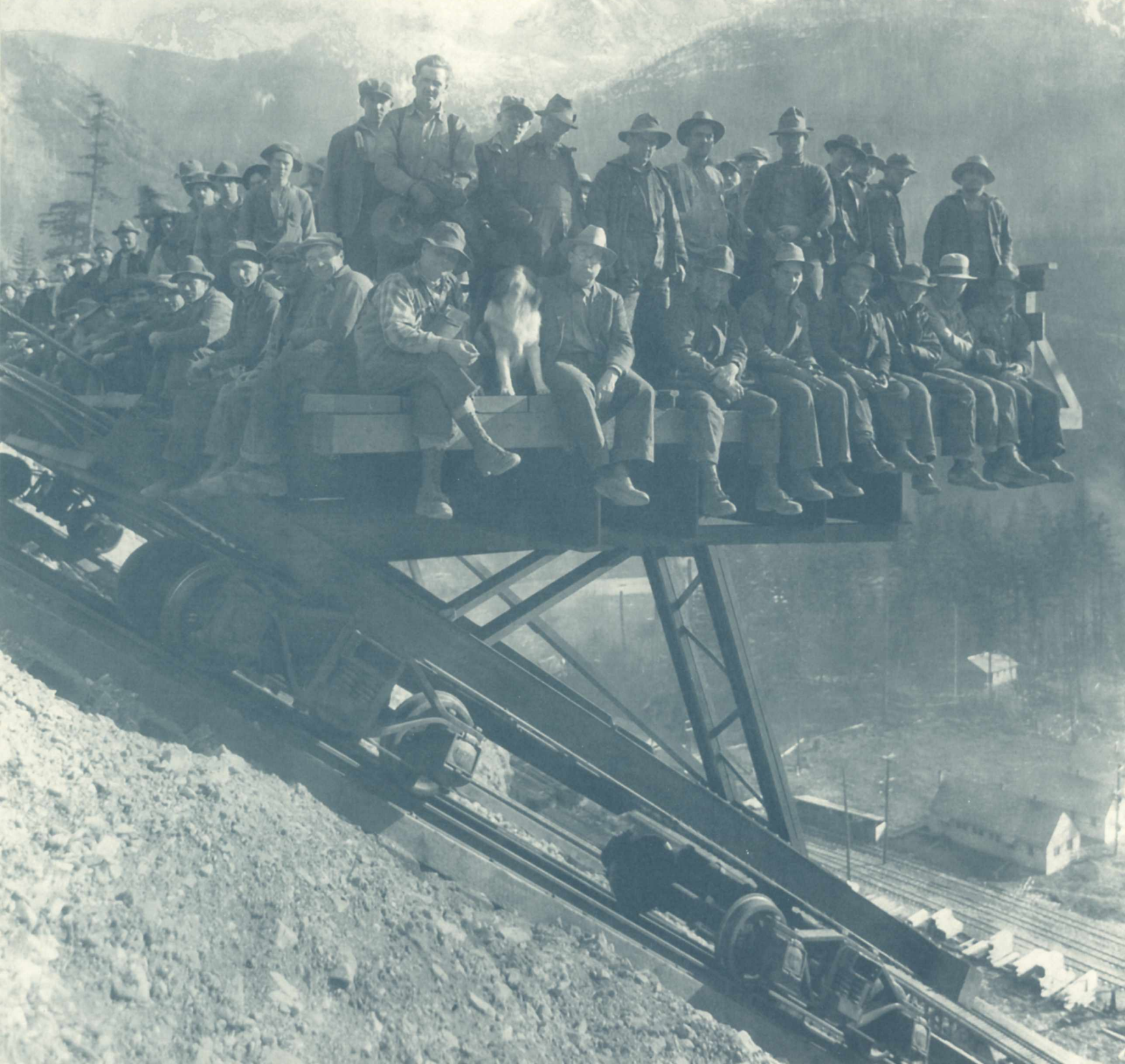
Incline railway at Diablo, used in construction of Diablo and Ross (originally Ruby Dam), designed as a permanent feature of the project (SCL-D-(28-4-14)-4).
