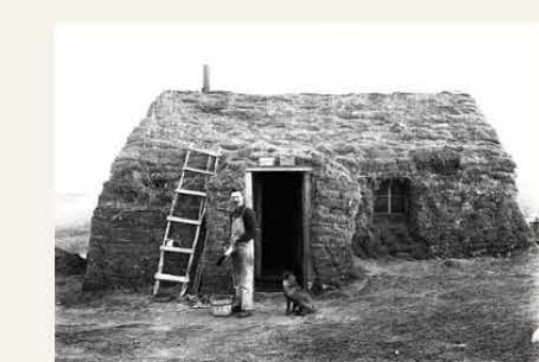
Blocks of sod cut from the deep topsoil of the grasslands were used by settlers to build temporary homes on the treeless plains of America's heartland. These "sodder" offered shelter from the intense heat or bitter cold until lumber could be imported from the
