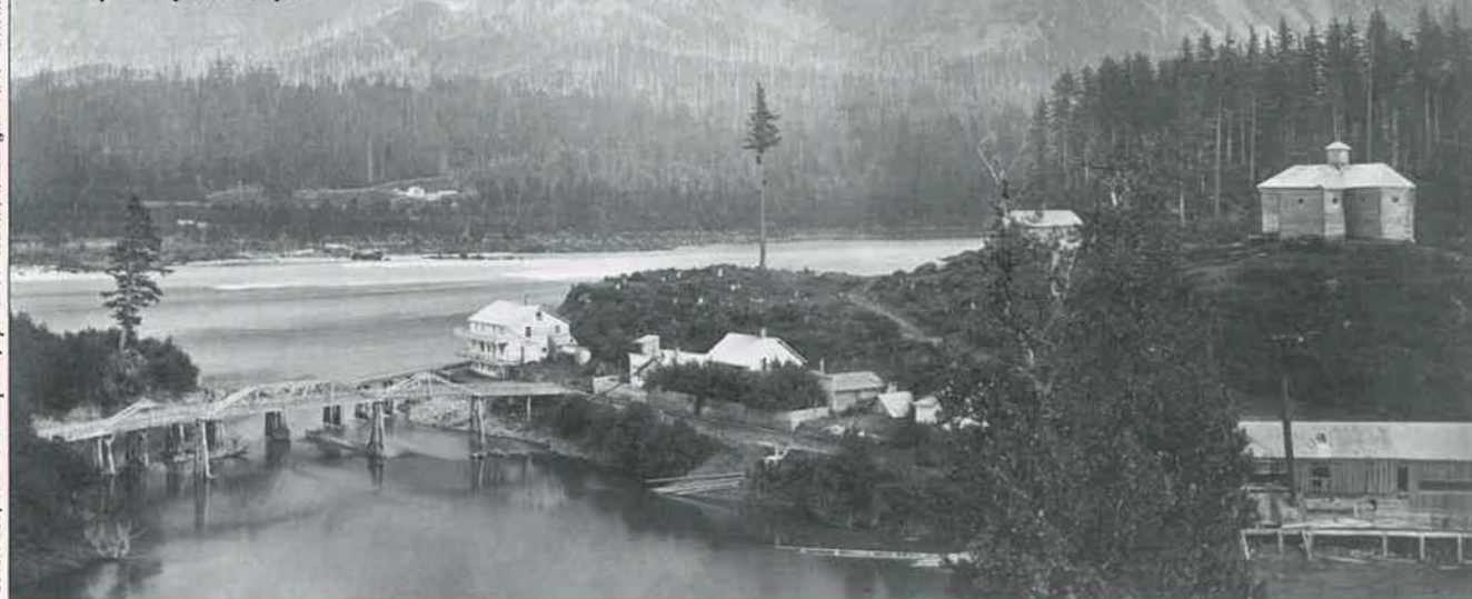
The upper Cascades of the Columbia River, 1867. The center building is the Bradford General Store; the mill where Willis Boatman obtained lumber is at bottom right. The large structure above the mill is Fort Lugenbeel, not yet built in 1852. The graveyard where Willis buried his brother lies in the wooded area just beyond the fort.
