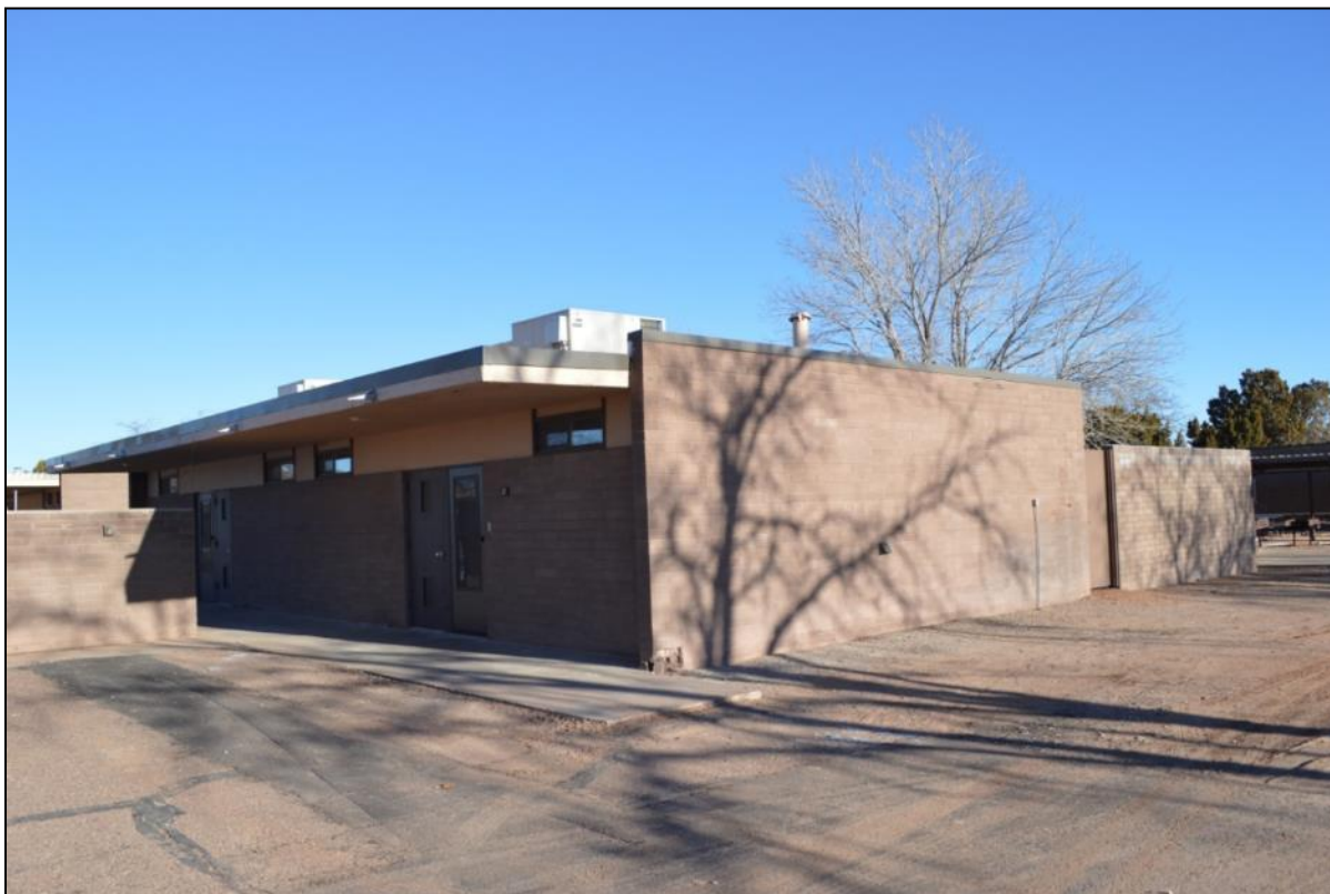
Photograph 30. Teacherage apartment (Resource 17).
