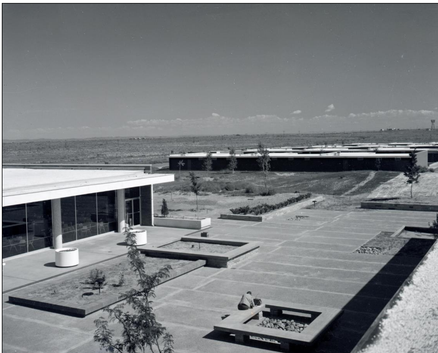
Figure 22. This ca. 1960s view from the roof of the apartment wings provides an overview of the central plaza, with the Painted Desert Oasis concession building to the left and the residence blocks in the distance, with block A the nearest. The area between the concession building and the residence block now holds the orientation loop. Courtesy Petrified Forest National Park, photographic archives, undated.
