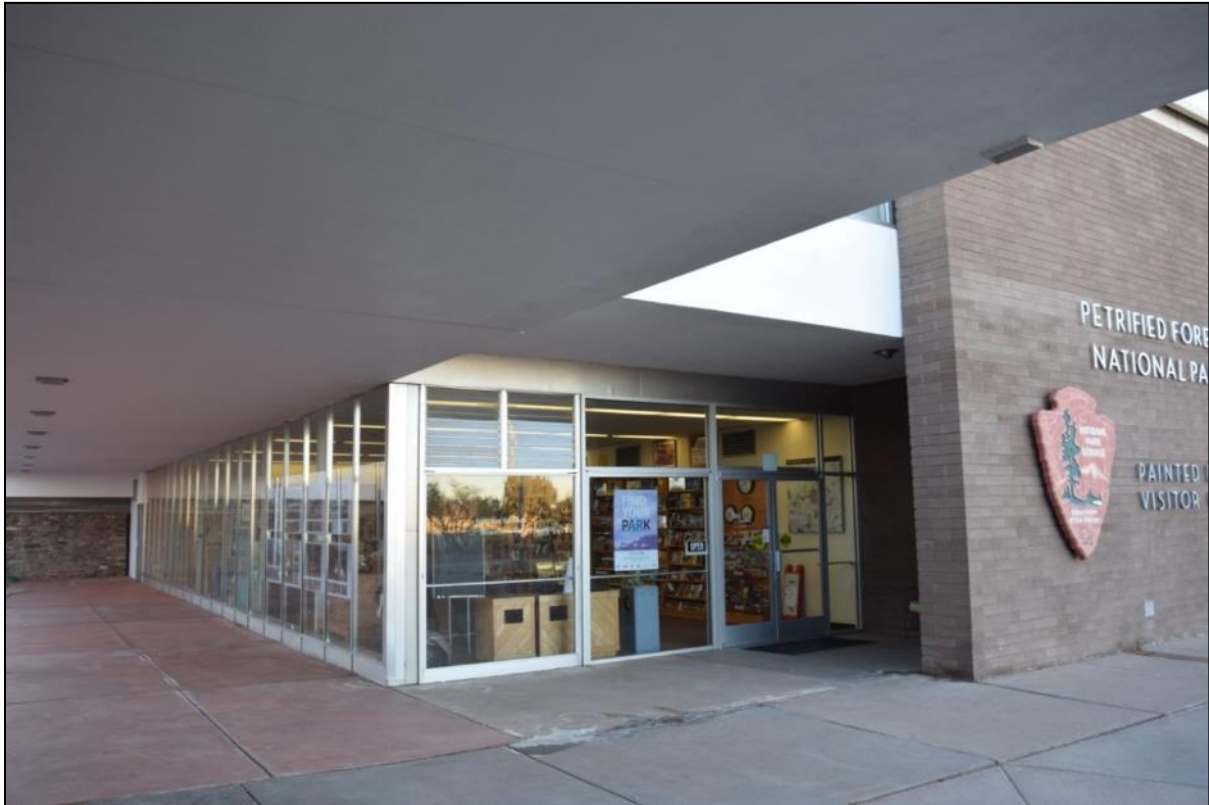
Photograph 3. Visitor center/administration building (Resource 1), entrance/lobby at northwest corner.
