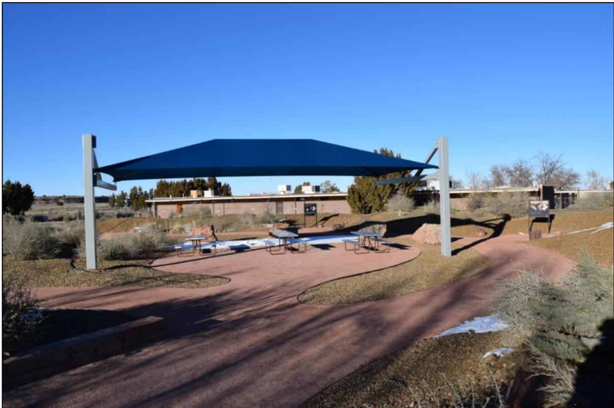
Photograph 16. Orientation loop (Resource 5), residence block A (Resource 13) in the background.
