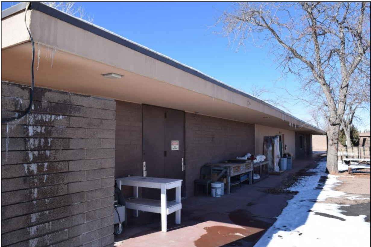
Photograph 36. Trailer court building (Resource 27), front (north wall).
