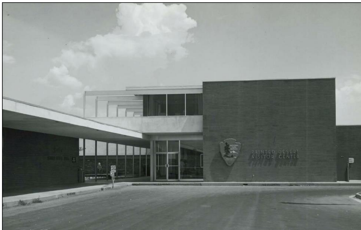
Figure 18. The visitor center/administration building is the focus of this 1963 photograph, with its glass curtain wall and second-story terrace with spider legs. The Painted Desert Oasis concession building is to the left. The apartment wing and plaza are visible in the opening between those two buildings. Courtesy Petrified Forest National Park, photographic archives, Philip Hyde, photographer, 1963.
