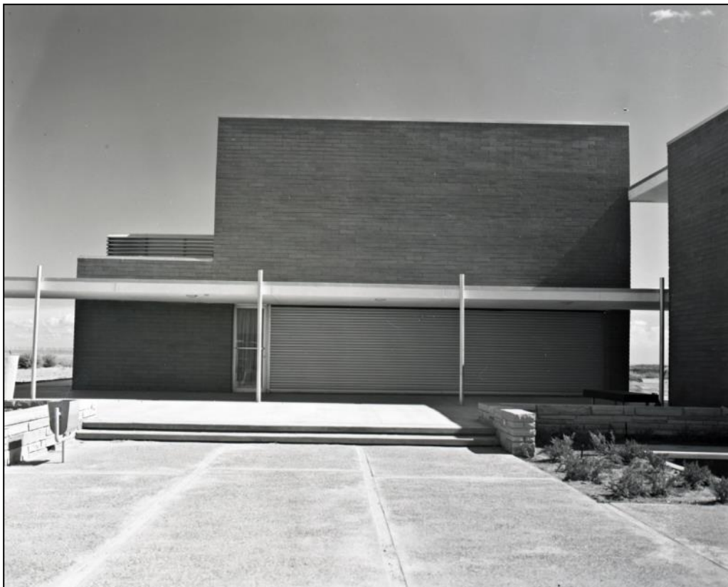
Figure 27. The front of the community building featured a wide roll-up door. The apartment wing is to the right. The Painted Desert School and the breezeway connector are not yet present on the left in this ca. 1963-64 view. Courtesy Petrified Forest National Park, photographic archives, undated.
