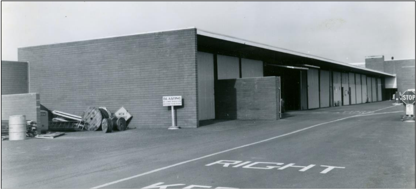
Figure 28. The long maintenance building lies at the west side of the maintenance yard with the visitor center/administration building in the distance to the right in this ca. 1960s image. Courtesy Petrified Forest National Park, photographic archives, undated.
