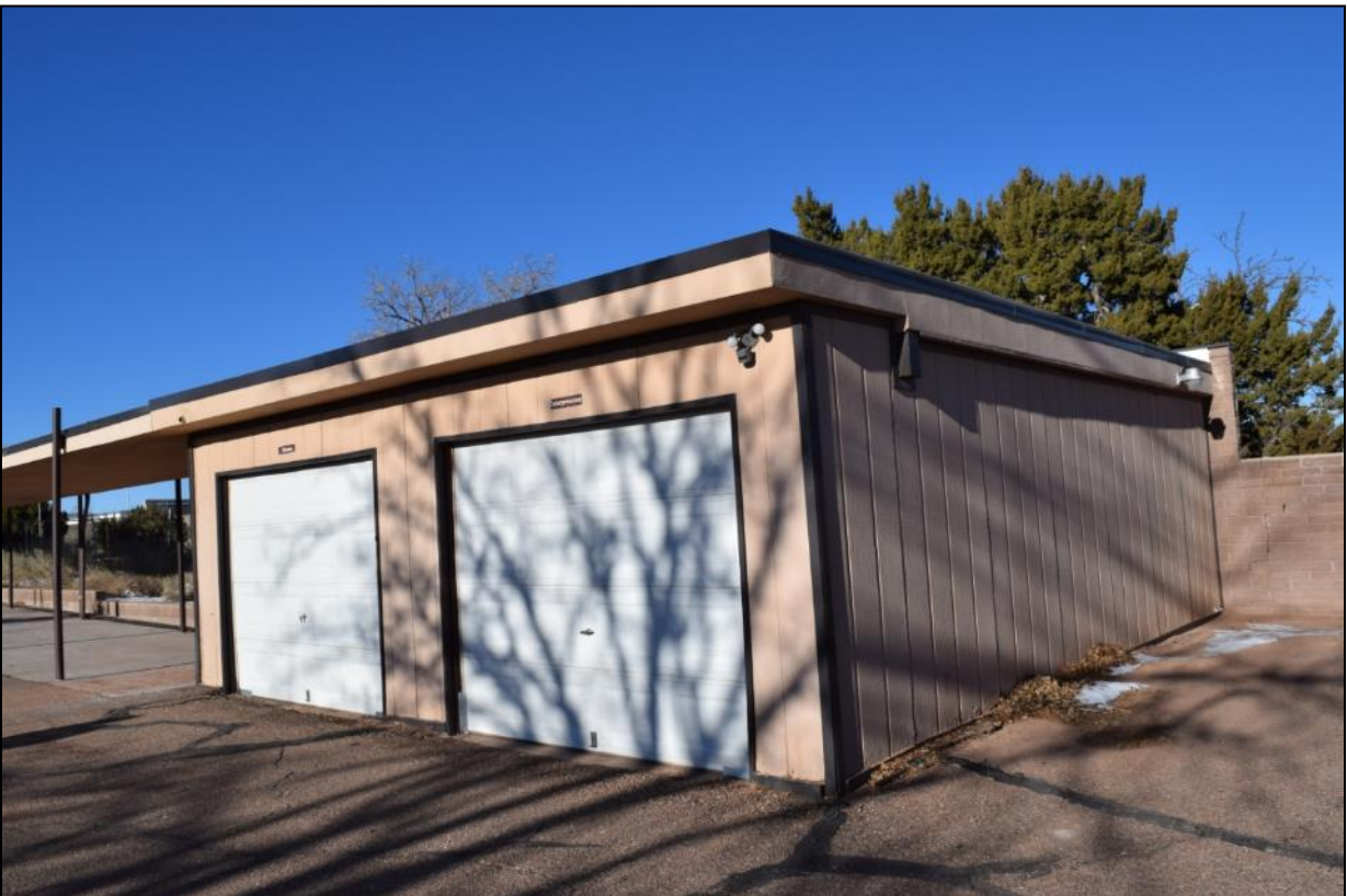
Photograph 32. Two-car carport (Resource 21) with covered walkway (Resource 6) to left.
