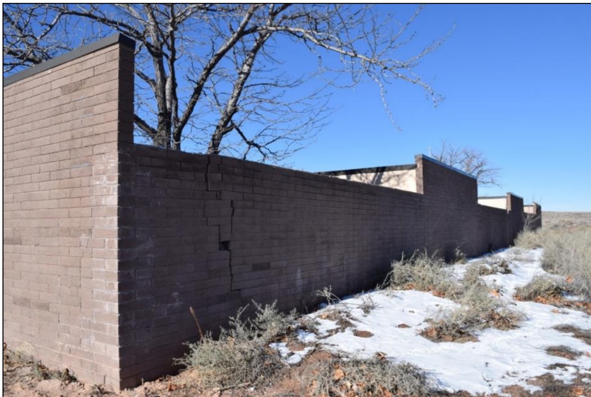
Photograph 29. Rear (north wall) of residence block D.
