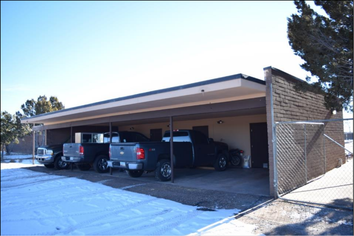
Photograph 31. Four-car carport (Resource 18), front (west) and south walls.
