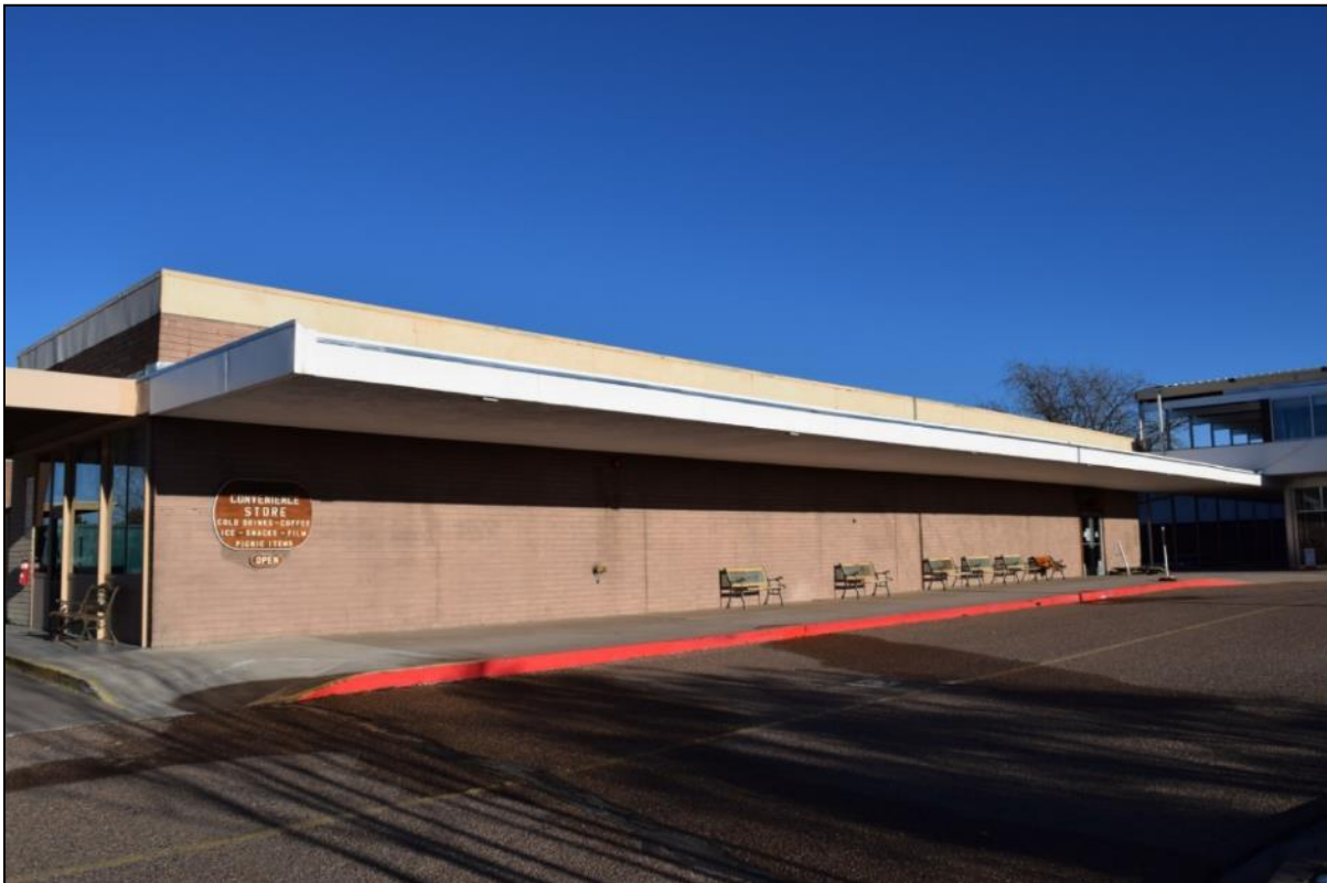
Photograph 8. Painted Desert Oasis concession building (Resource 2), south wall.
