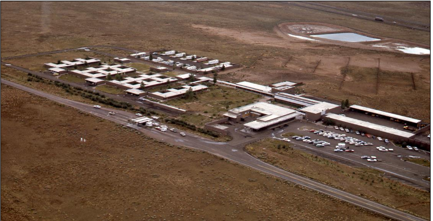
Figure 17. This oblique aerial view east shows the complex ca. 1968-70. Interstate 40 and sewage lagoons are in the upper right, and the park access road crosses diagonally in the lower part of the image. The visitor center/administration building is the taller building at the corner of the parking lot. The angle of the photograph gives a good perspective on the nature of the courtyards within the residence blocks (the four large buildings in the left center of the image). Courtesy Petrified Forest National Park, photographic archives, undated.
