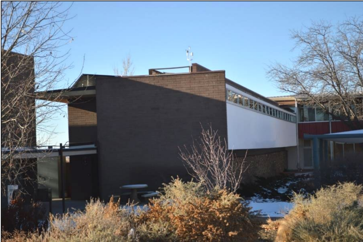
Photograph 11. Apartment wing (Resource 3), north and west wall. Visitor center/administration building is to the right.
