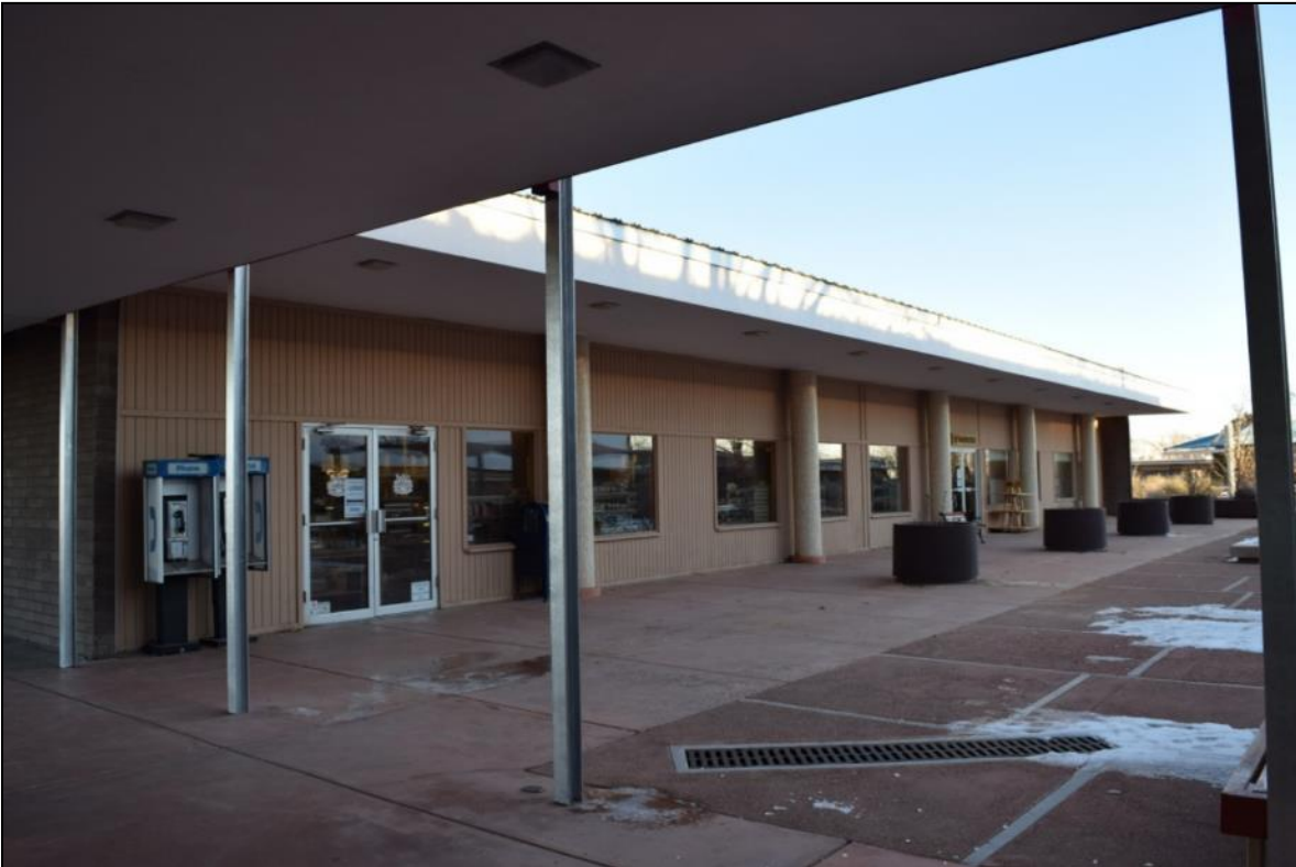
Photograph 7. Painted Desert Oasis concession building (Resource 2), front (east wall). Note columns clad with tile.
