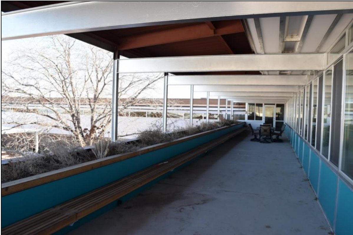
Photograph 5. Visitor center/administration building (Resource 1), north terrace (second story).
