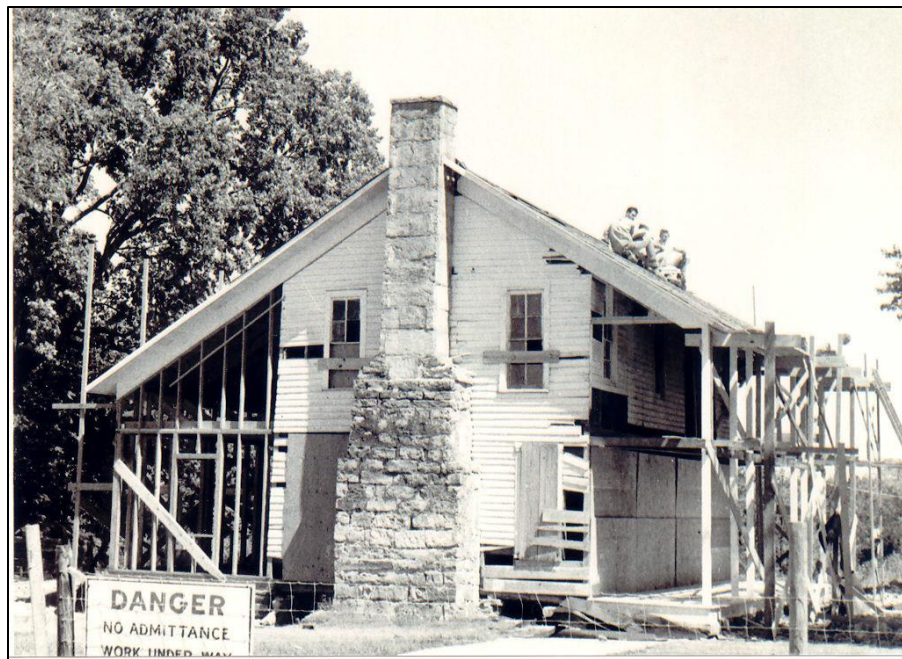
Figure 30. The Elkhorn Tavern undergoing historic restoration. Pea Ridge National Military Park.
