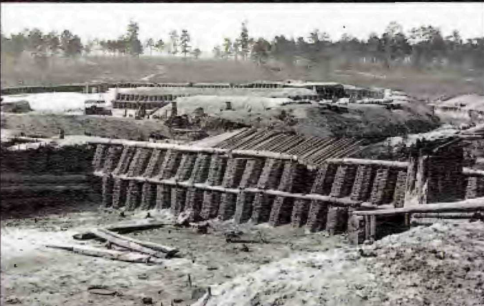
Fort Sedgwick earned the nickname "Fort Hell" because its close proximity to Confederate batteries made it a prominent target. The wickerware (gabions) helped protect the position.
