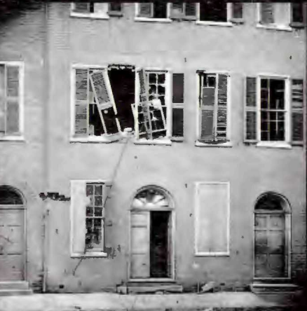
This townhouse on Bollingbrook Street was one of many houses damaged or destroyed by Union shot and shell during the siege.
