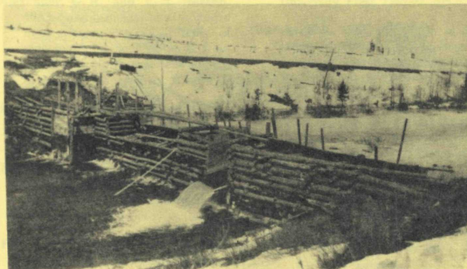
Figure 2: Logging dam typical of the type constructed at the mouth of Beaver Creek around 1905. Earthen materials may have been more important in construction of the wings of the Beaver Creek Dam.
