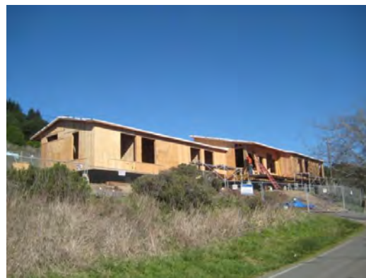
A current look at the new hostel building under construction.
