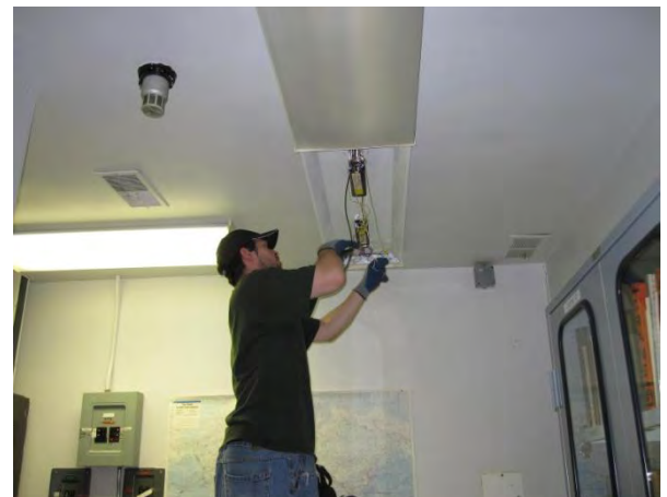
Smart Lights changing out ballasts at NDOC.
