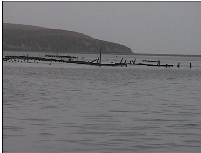
Dilapidated oyster racks within Drakes Estero.
