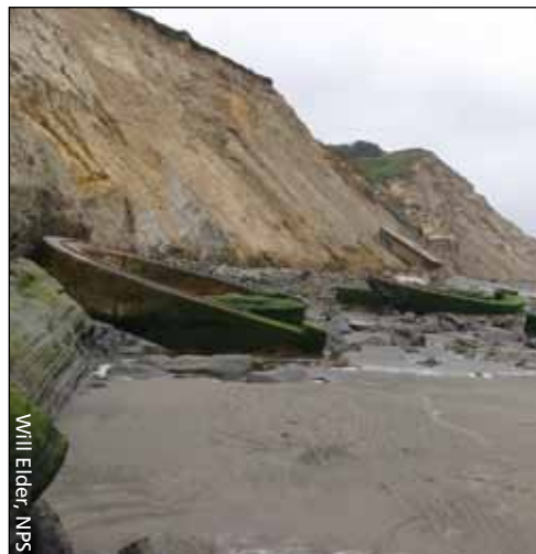
Already erosion-prone cliffs at Fort Funston will disappear even faster as a result of rising sea levels and fiercer storms
