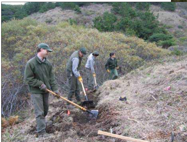
Crew working on Muddy Hollow Trail
