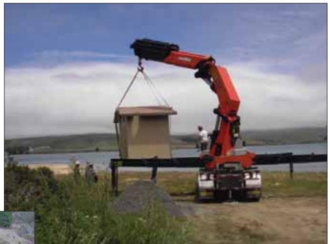
Lowering of restroom at Tomales Bay Beach
