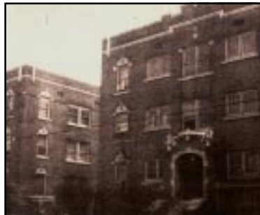
Historic pictorial evidence shows the original multi-pane configuration of the windows.
