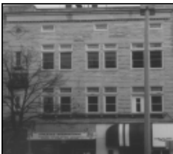
Before and after rehabilitation, one-over-one sash helped retain this commercial building's historic character.
