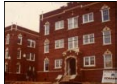
After rehabilitation the new multi-paned sash are appropriate to the historic style and character of the apartment buildings.
