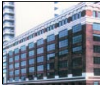
Installing multi-pane steel sash helped restore the building's historic appearance.
