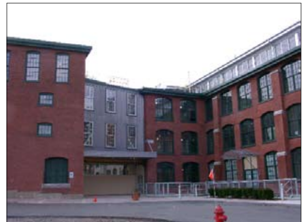
Introducing a three-story glass wall as seen above in the drawing, would have altered the character of the bridge and did not meet the Standards. A more compatible treatment was approved where existing window openings were retained and a metal corrugated wall membrane and simple canopy were added (bottom).
