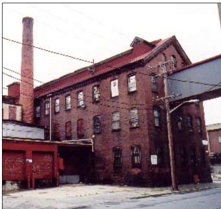
Industrial building and bridge before rehabilitation.
