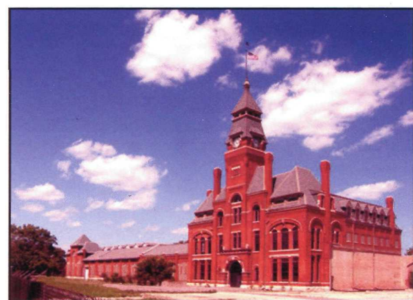
Pullman National Historical Park Visitor Center
