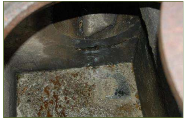
Storm drain filled with vegetable oil fuel mixture.
