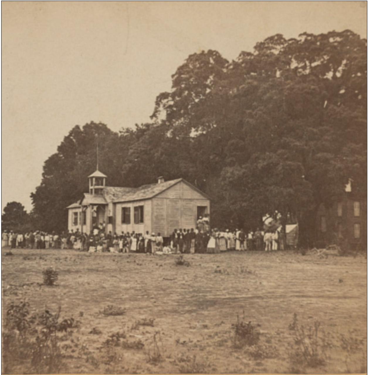
Figure 6. Prefabricated Penn School Building
