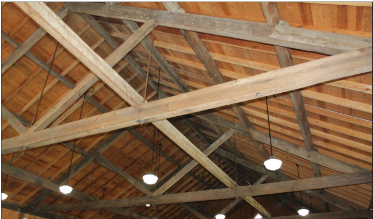
B. Roof Structure
