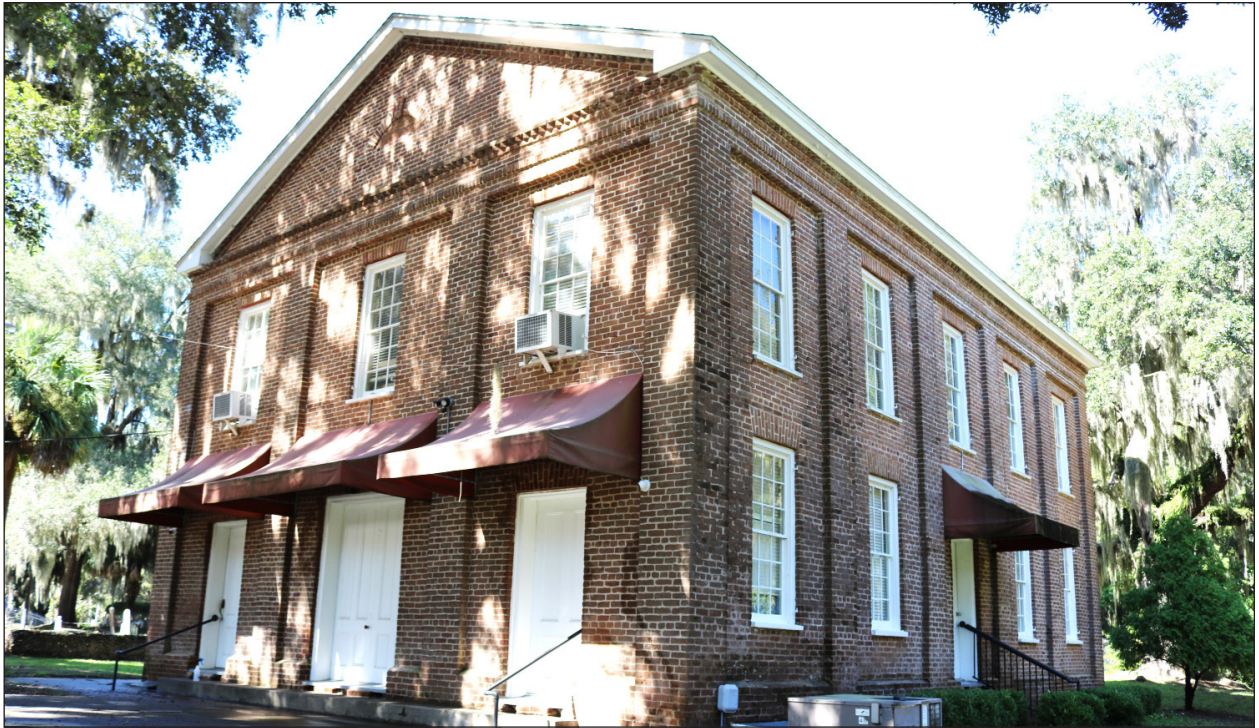
A. Northeast Oblique, Looking Southwest
