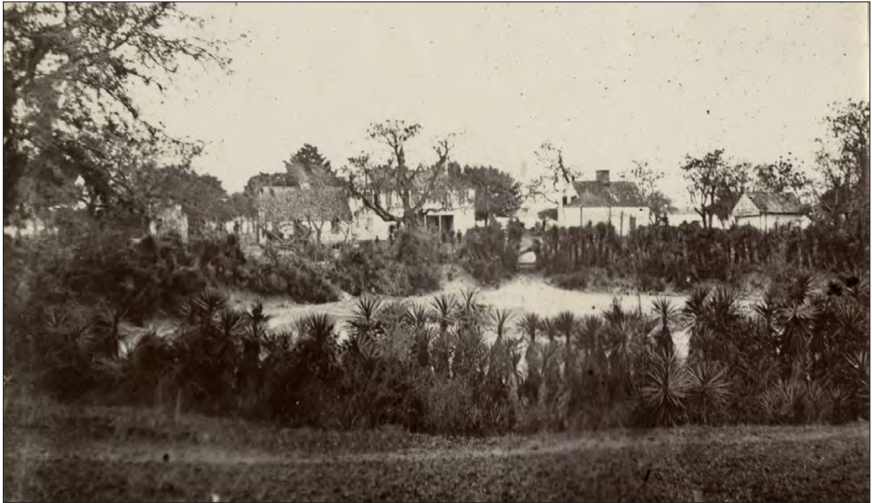
Figure 41. 1863 Photograph of Sink Hole
