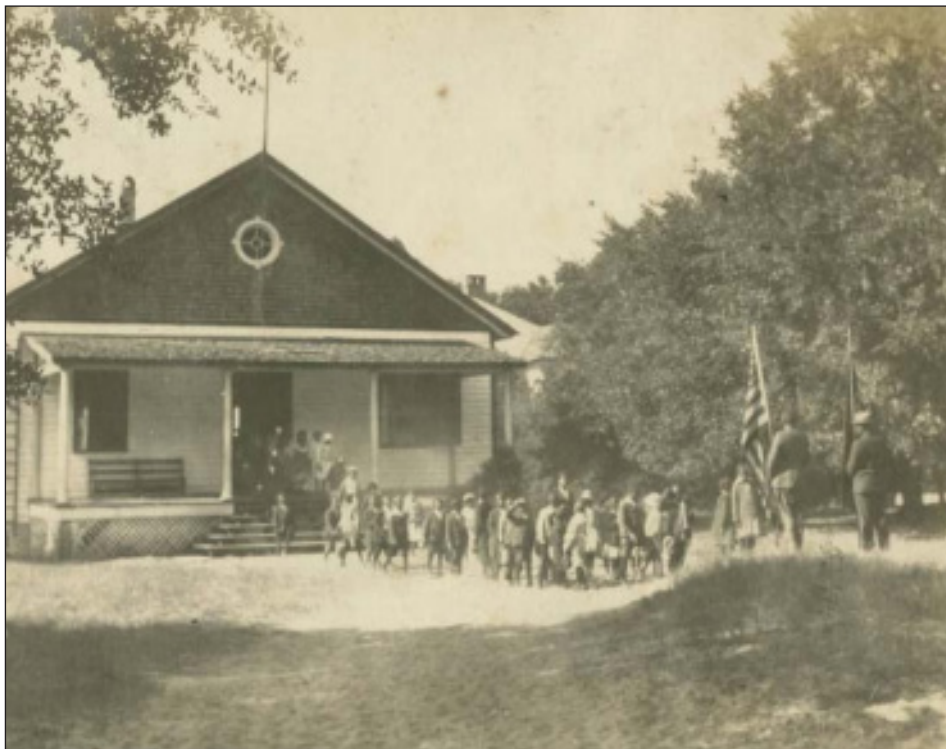
B. Historic Photograph of Darrah Hall Circular Window Source:Image 04596lb: Leaving Darrah Hall, Penn School Papers #3615, No Date.
