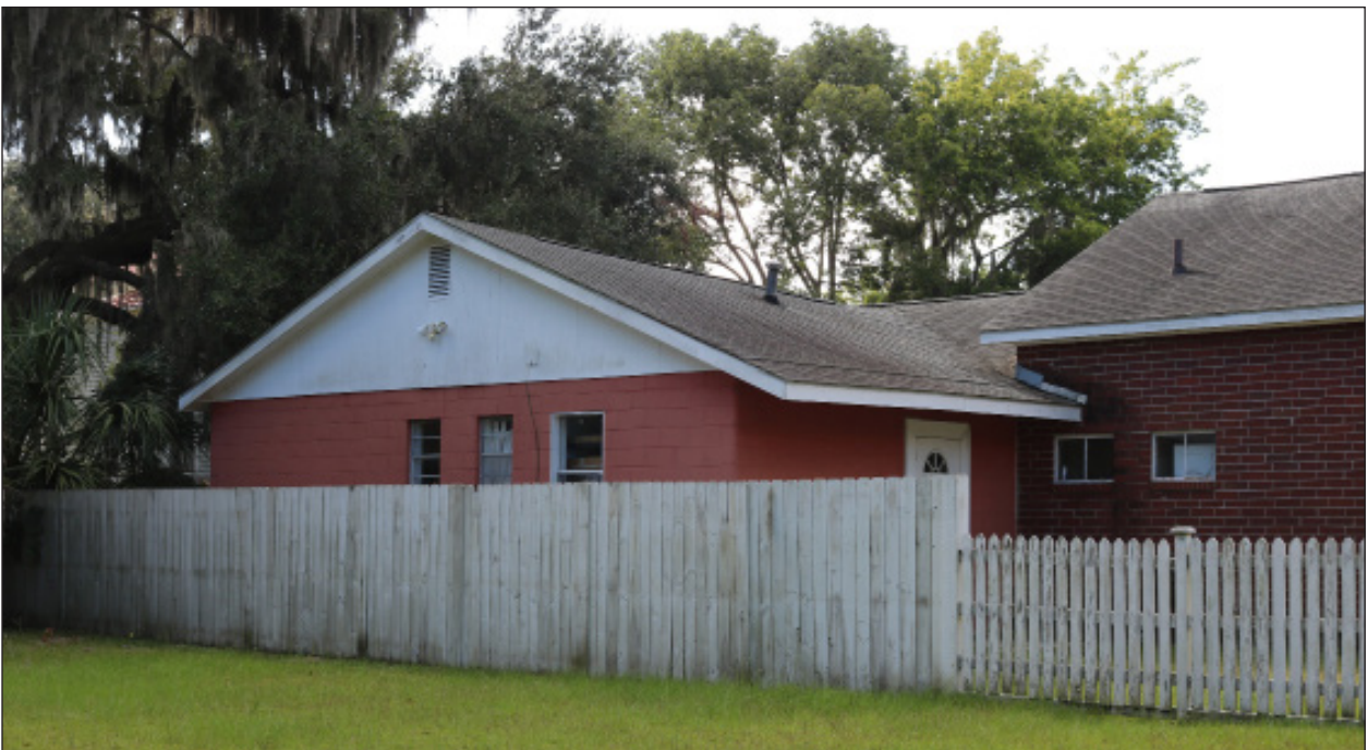
B. Addition on North Elevation, Looking South
