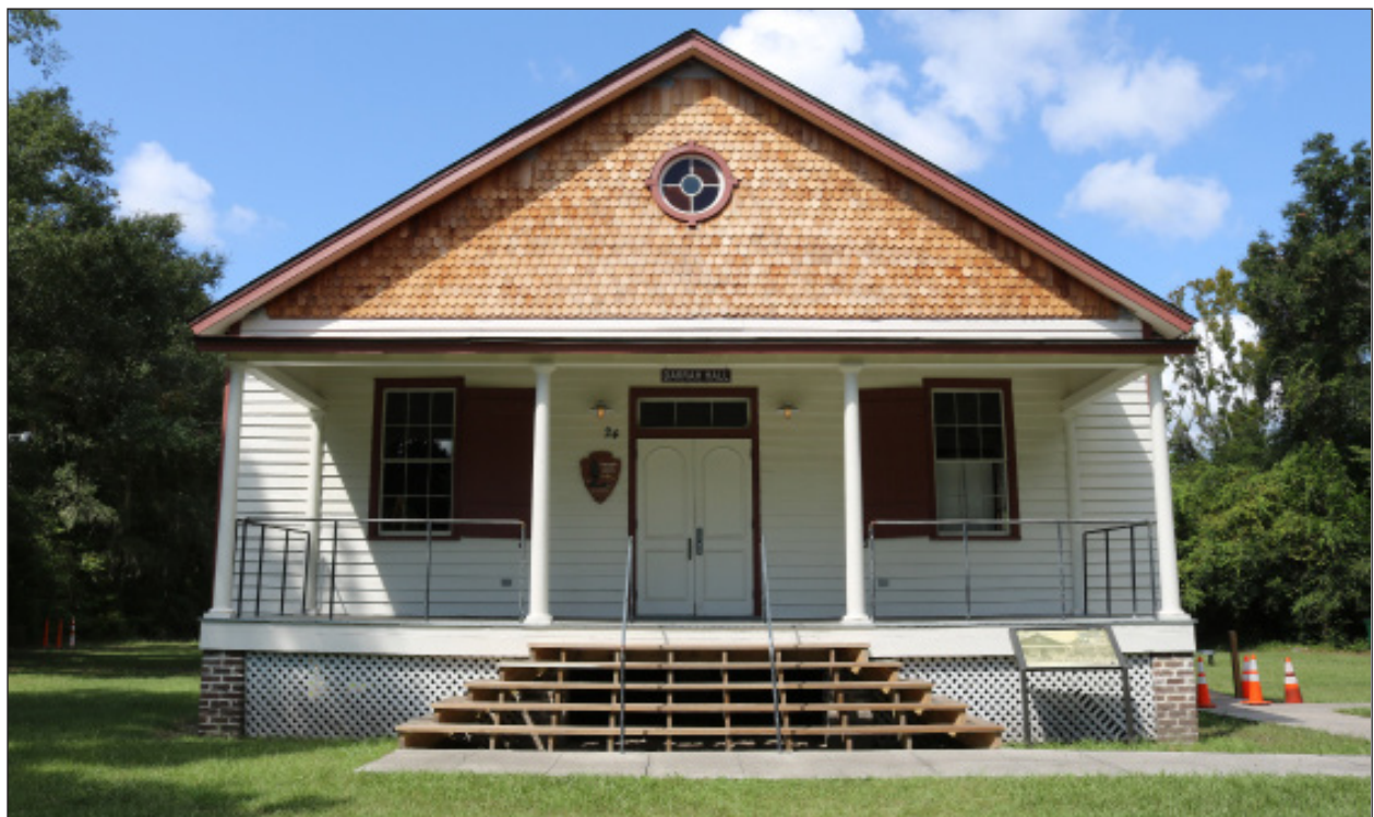
B. Façade, Looking West
