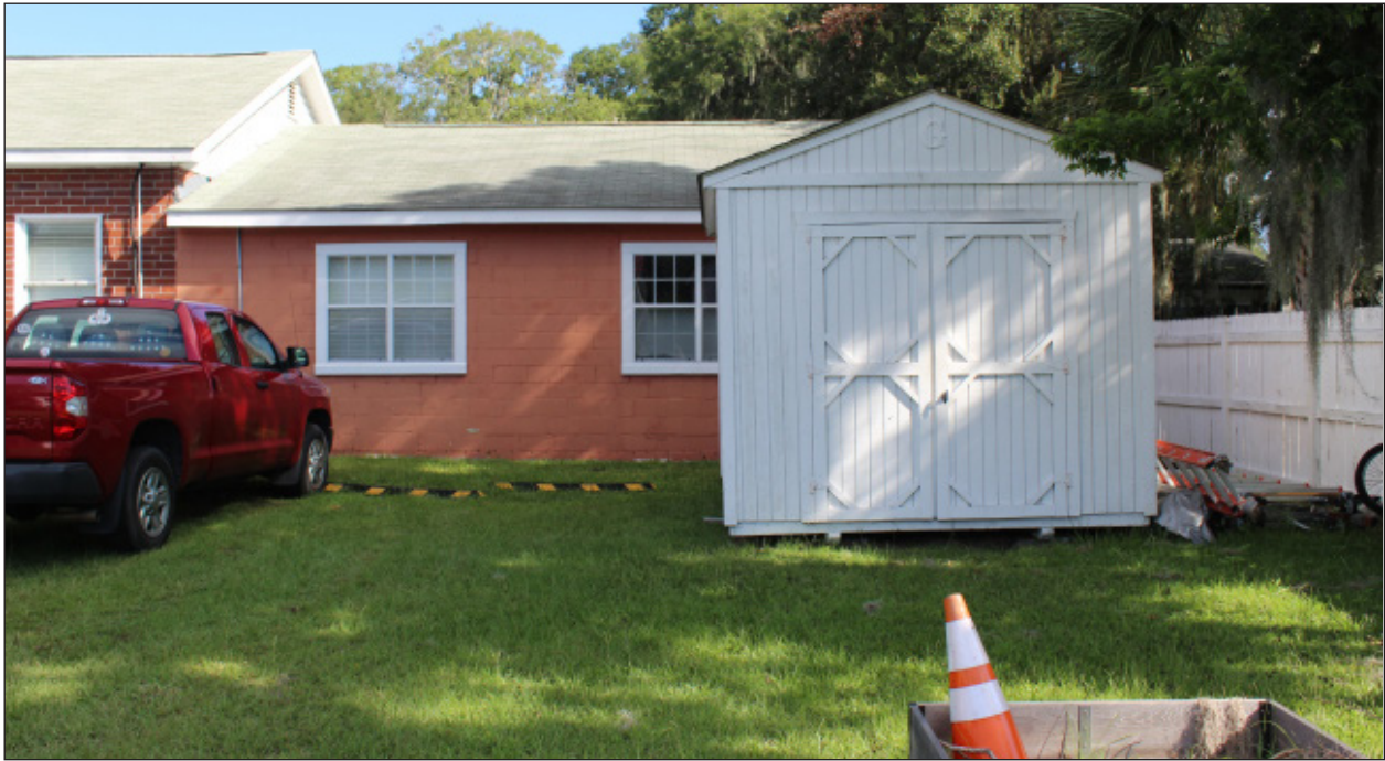
A. Rear Addition, Looking North
