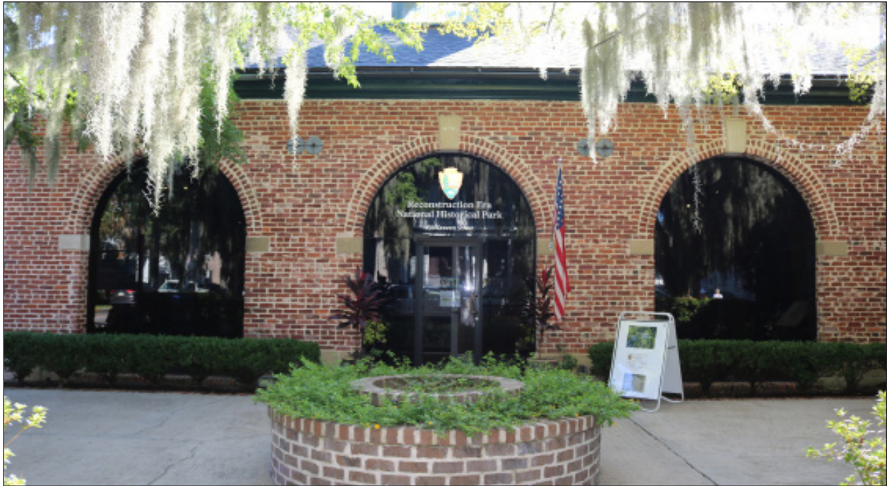
A. West Elevation and Front Entrance, Looking East
