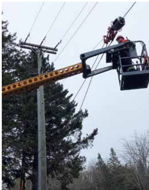
Fibre-optic cable was laid through the spring and summer of 2021.
