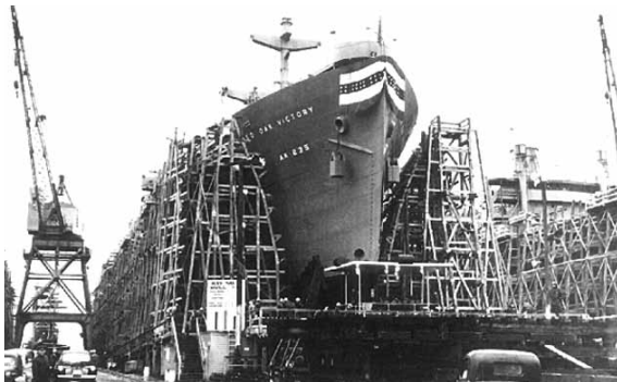
The SS Red Oak Victory being constructed, Richmond Museum of History Collection.
