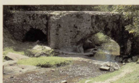
The arches of the two-centuries-old Espada Aqueduct.
