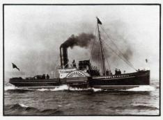
Eppleton Hall Built in England in 1914, Eppleton Hall is reminiscent of the paddle tugs that towed ships into San Francisco Bay during Gold Rush times. The tug's side-lever steam engines are descendants of engines used in sidewheel steamers that connected San Francisco to Panama.
