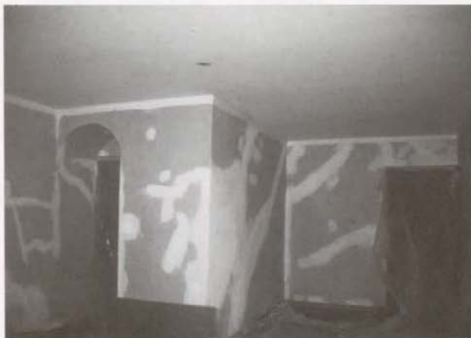
Alice's Room: After Restoration (plaster repaired, ready for wallpapering).
