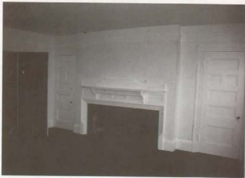
South Bedroom: After Restoration (ready for wallapering).
