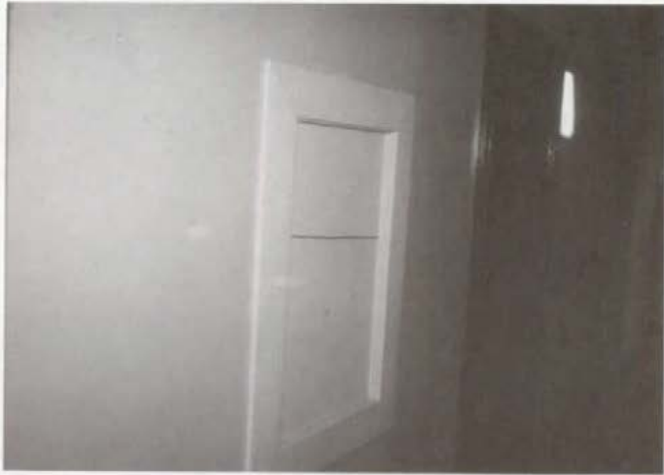
Typical Firebox Location in Hallway: Before Restoration
