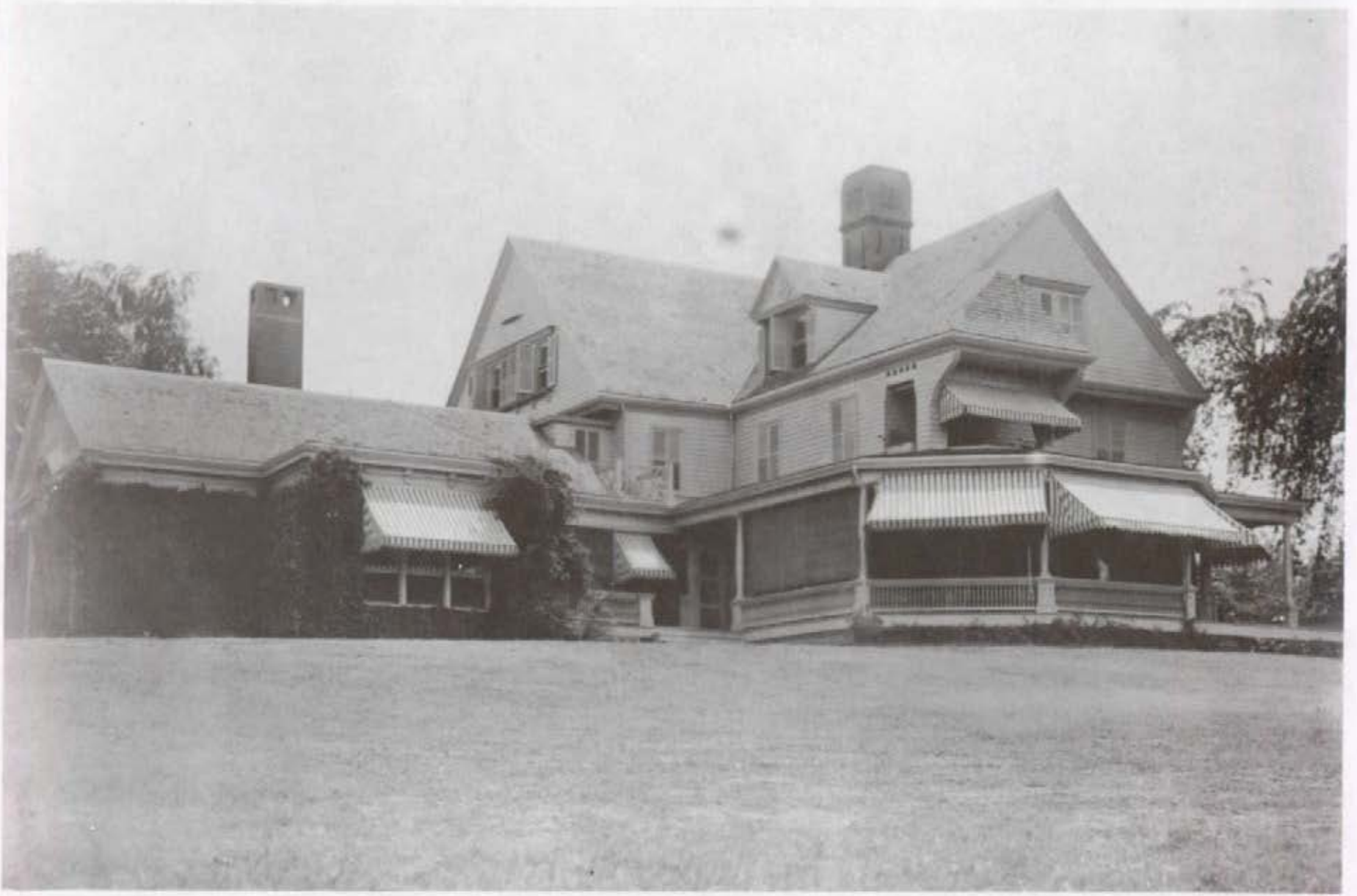
Figure 16. View of west elevation, 1907.
