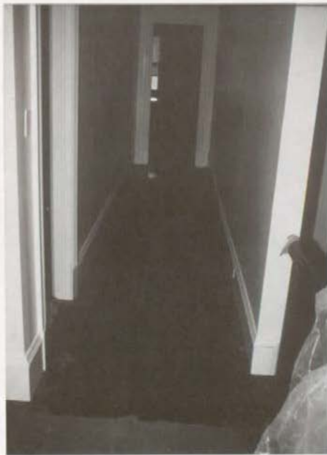
Third Floor Hall: After Repainting
