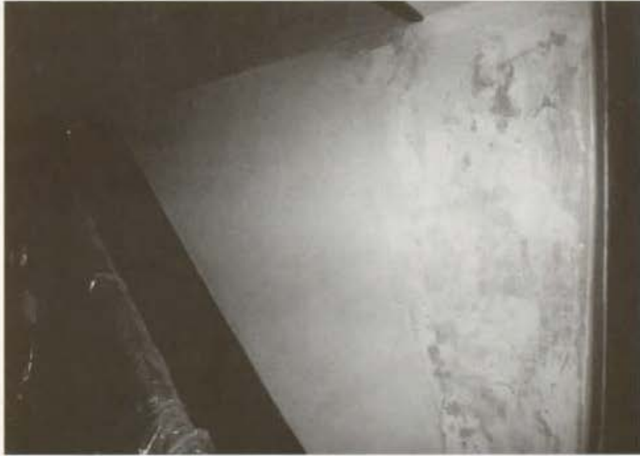
Second Floor Rear Hall Stairway: After Replastering
