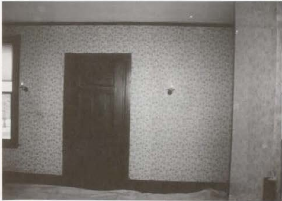
Nursery: Before Restoration
