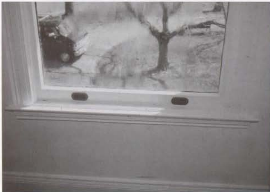
Typical Window Sash Condition After Restoration
