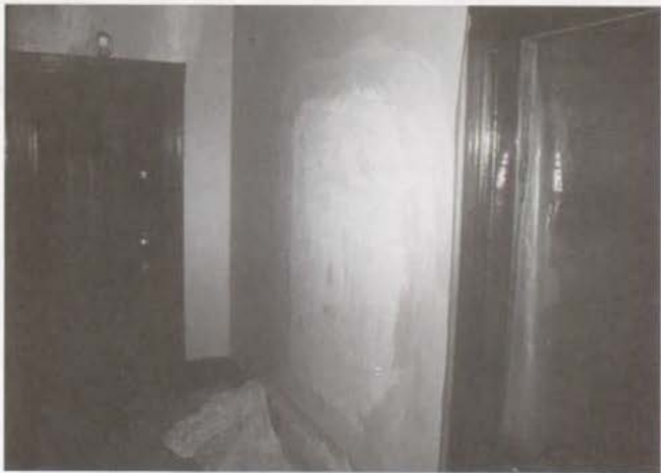
Typical Firebox Location After Removal and Replastering
