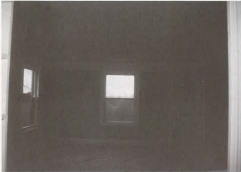
Gate Room: After Restoration
