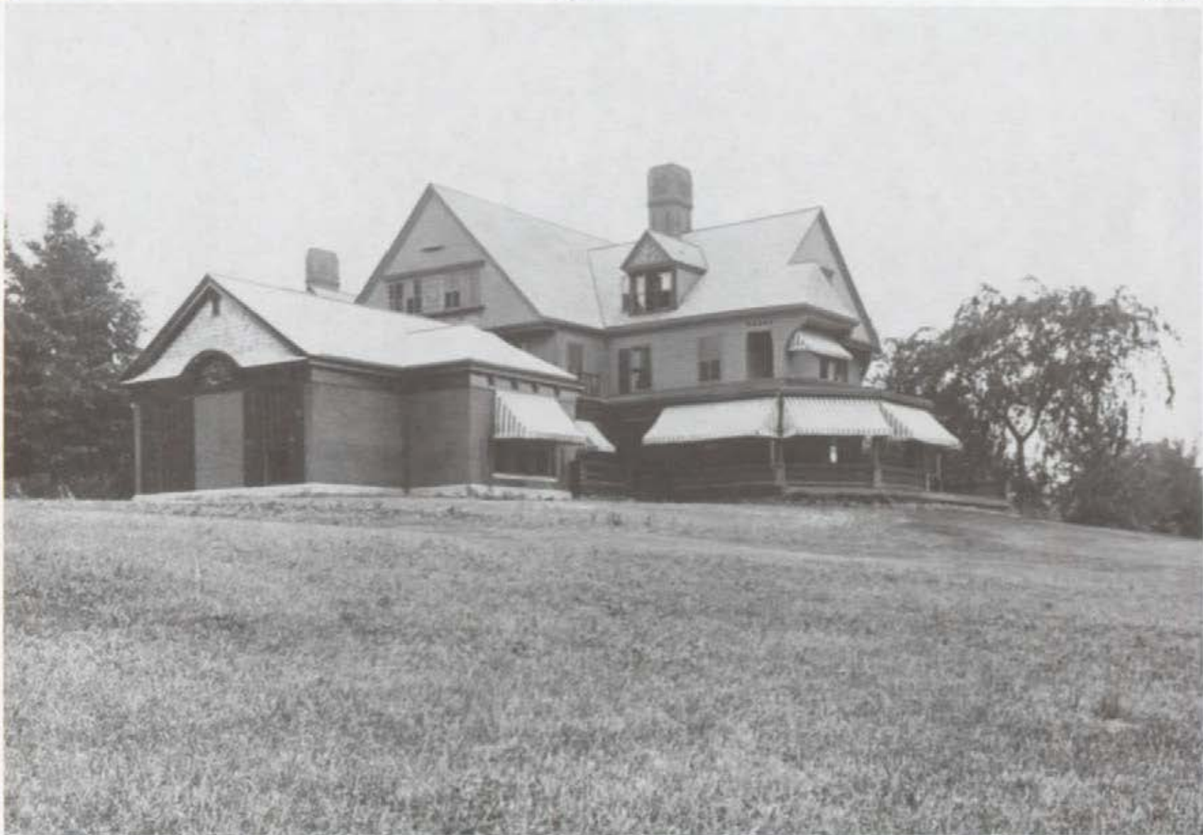
Figure 11. North and west elevations after completion of north wing (Trophy Room), 1905.
