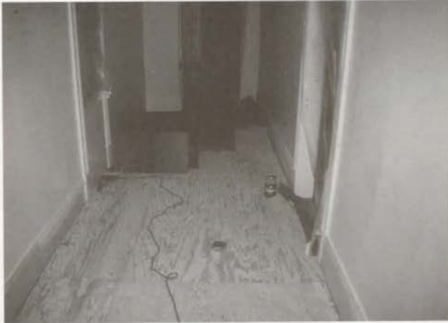
Third Floor Hall: Plywood Installed On Floor
