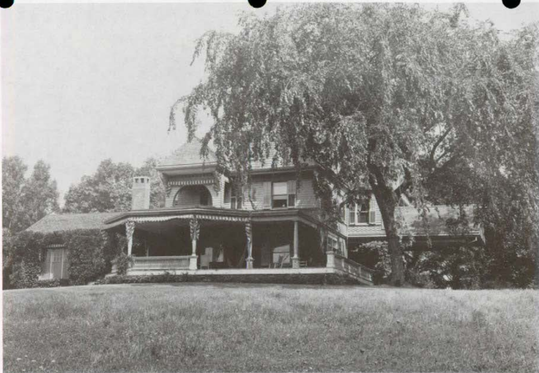
Figure 17. Direct view of west elevation, 1907.
