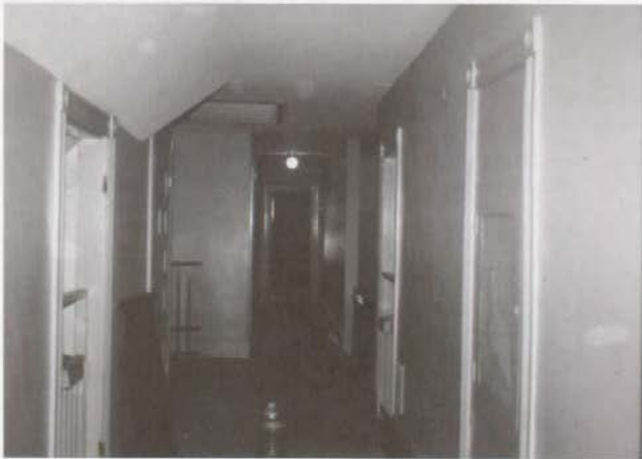
Third Floor Hall: Before Restoration
