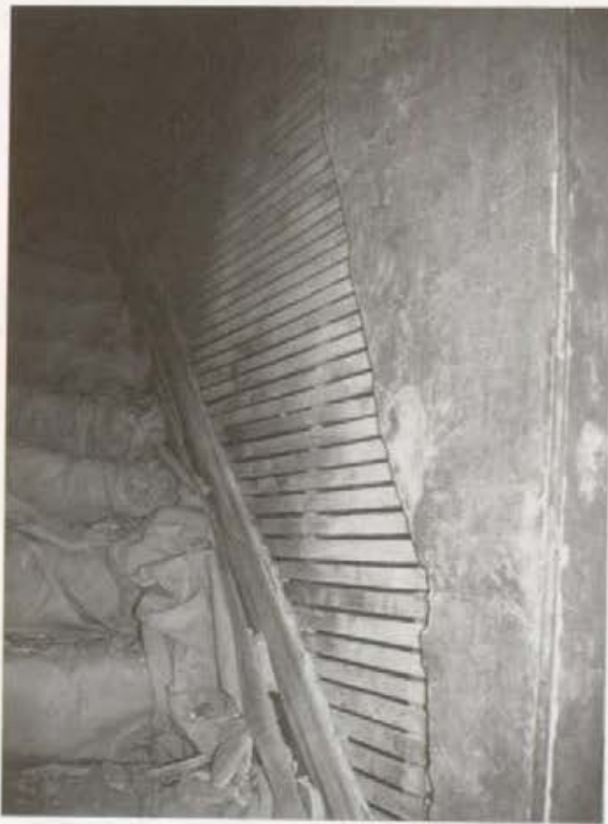
Second Floor Rear Hall Stairway: During Restoration (plaster removed)
