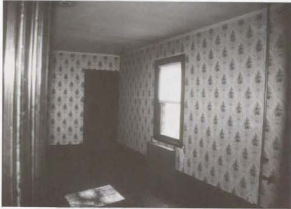
Alice's Room: Before Restoration
