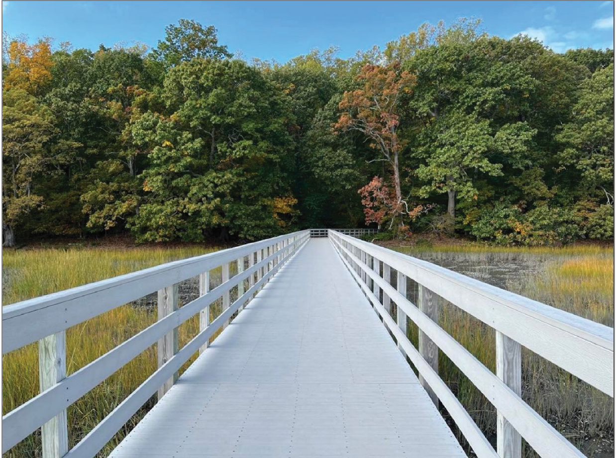
Figure 16. Photograph of the reconstructed nature trail boardwalk following Hurricane Sandy. View of the boardwalk is facing north across the Eel Creek wetland and adjoining forested uplands of the historic site. Reconstruction of the new boardwalk was completed in early 2014 using recycled composite decking with an improved substructure. (NPS/MARIE C. CLIFFORD).
