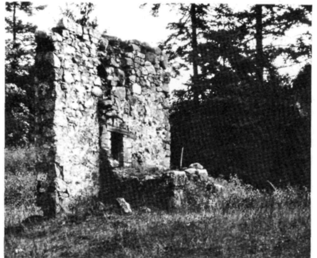
Remains of stone work at Blacksmith Shop, English Camp.
