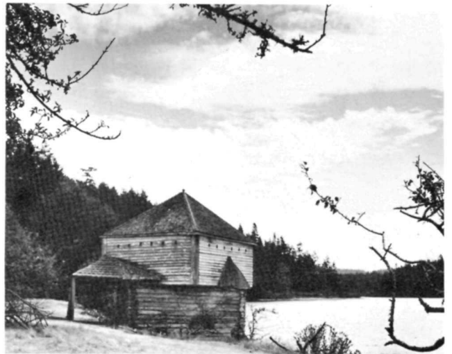
Blockhouse at English Camp looking southeast along the shore of Garrison Bay. The best preserved of historic structures on the island, it served the British during their 13-year occupation of San Juan Island.
