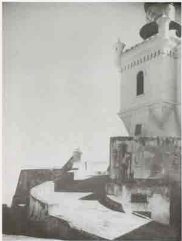
Figure 28. Hi Morro, lighthouse. (Photo by J. Boucher, 1962. NARS 16616.)
