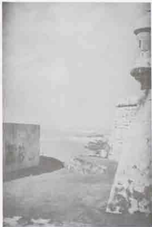
Figure 1. Austria Bastion, south salient angle. (Photo by T.T. Waterman, 1938. HABS, PB 7-0470 4-0, PB 88, 16614.)
