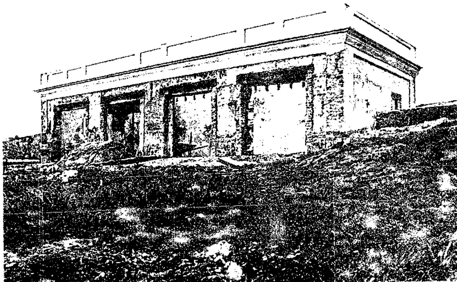
Figure 17.8. North and west elevations of the Guardhouse in the process of restoration, October 29, 1981. (San Juan NHS Archives.)
