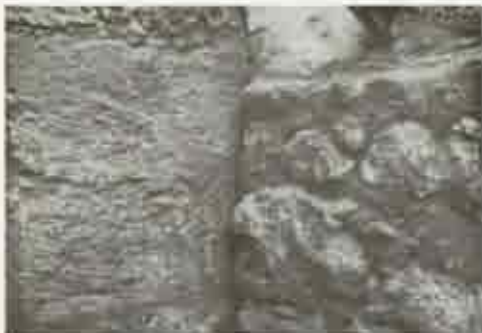
Figure 9. Rubble wall (ca. 1771) meeting seventeenth-century orillon corner. (Photo by E.S. Cliver, 1990.)
