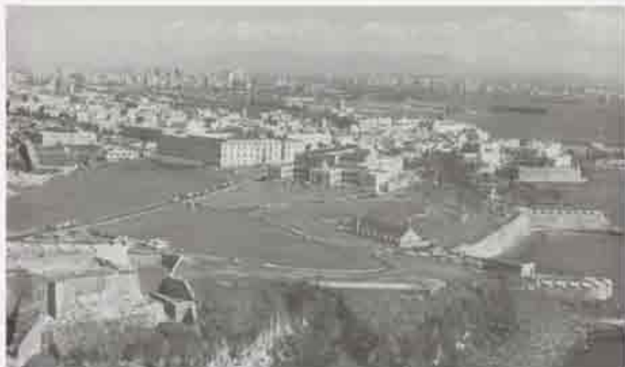
Figure 12. East view, 1988. Aerial view from el Morro toward the city showing the paved road system, 40-car parking lot; parallel parking, the Dutch Monument, tennis courts, the chain-link fence, and the play area in Parcel 9. PRMPO, San Juan, PR.
