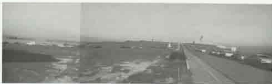
Figure 19. Composite photograph, West View, 1991 (View 3). Vista from intersection of Mahlonie and el Morro Roads shows el Morro, Dutch Monument, parking, and Powder Magazine area. Photography by Richard C. Criscon.
