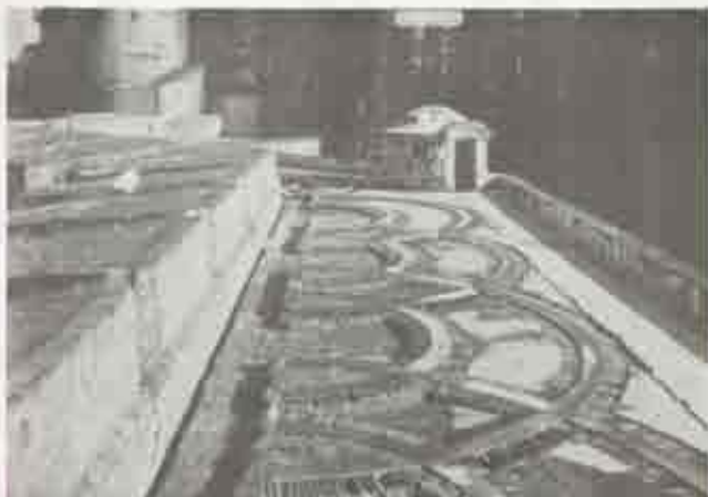
Figure 27. Tracks for 1860's gun emplacements on Santa Barbara Bastion. (J. Soucher, N332, 1960.)
