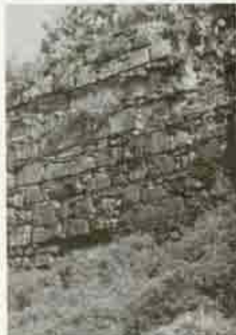
Figure 15. Remains of seventeenth c. retaining wall at the sea end of the counterscarp. (E.S. Cliver, 1890.)
