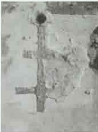
Figure 31. Double cross imprint in the casemate wall plaster, possibly from a bracket. (S.S. Cliver, 1992.)
