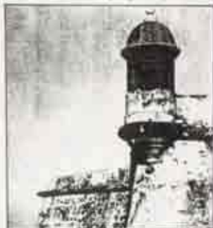
Figure 34. Rebuilt sentry box on Austria Bastion. (J. Boucher, NABD, 1940.)
