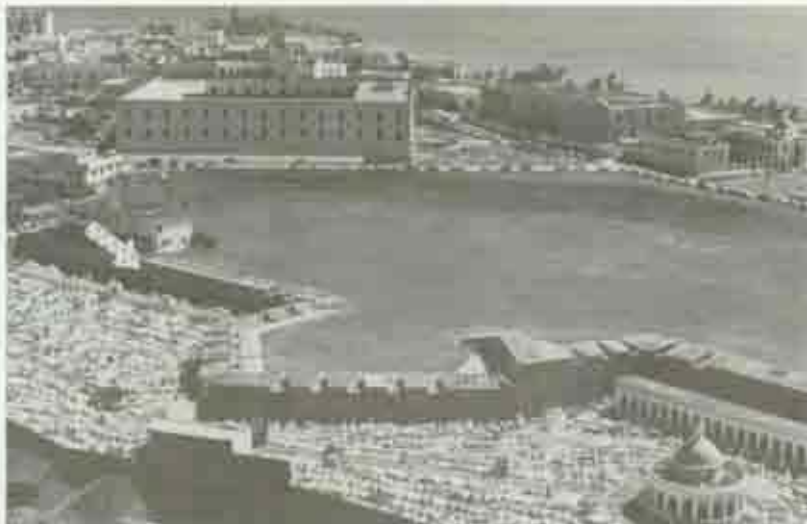
Figure 34. North wall - Santa Domingo to the left, Santa Rosa Bastion at center, cemetery in foreground, Calleja Barranca and city in background. Arrow indicates tunnel to the cemetery. (HSDO, San Juan, 1955.)
