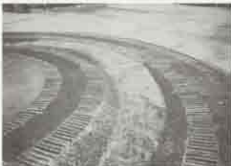
Figure 24. Tracks for an 1850's gun emplacement; note groove in dark stone from the iron rail. (Photo by S.R. Clivar, 1988.)
