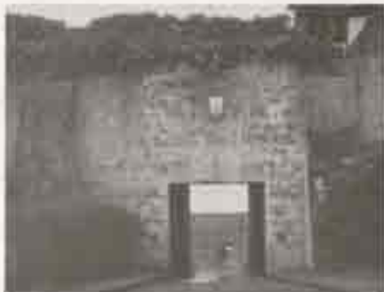
Figure 8. San Juan Gate, east elevation from Recinto Oeste. (Photo by E. Crismon, 1996.)
