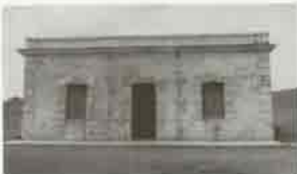
Figure 23. San Antonio Guardhouse at San Antonio Bastion. (Photo by E. Crisson, 1980.)
