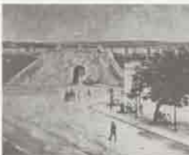
Figure 10. West elevation of Puerta de Santiago, ca. 1890. Photo by Feliciano Alonso. (Repro. in A.M. Rivera, 1989.)
