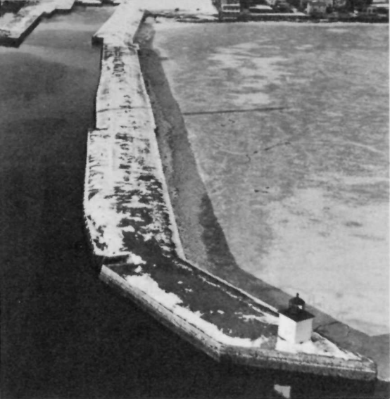
Derby Wharf with Central Wharf in upper left the structure in 1801 and completed it in its present form.
