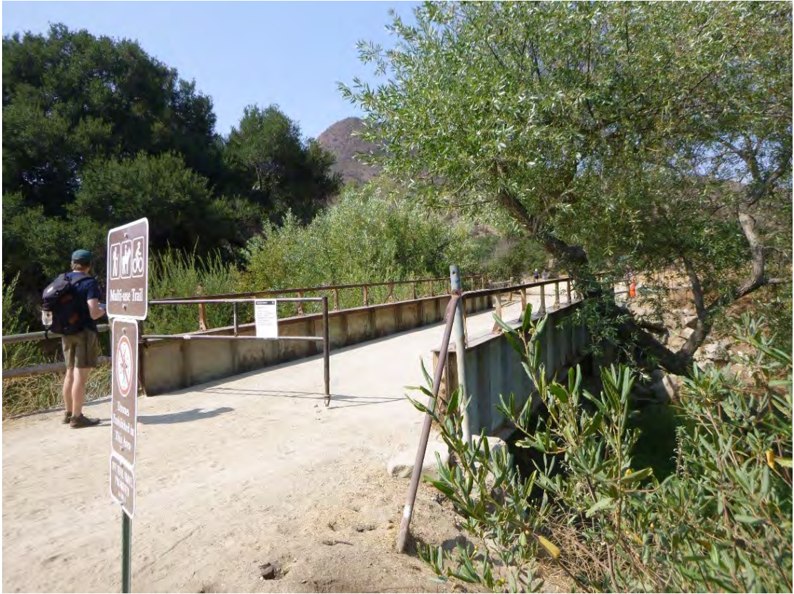
Buildings and Structures 4: Medea Creek Bridge, looking southwest (NPS, August 2021).
