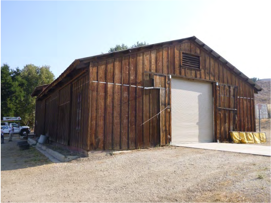
Buildings and Structures 2: Mill/carpenter shop building, south elevation (NPS, August 2021).
