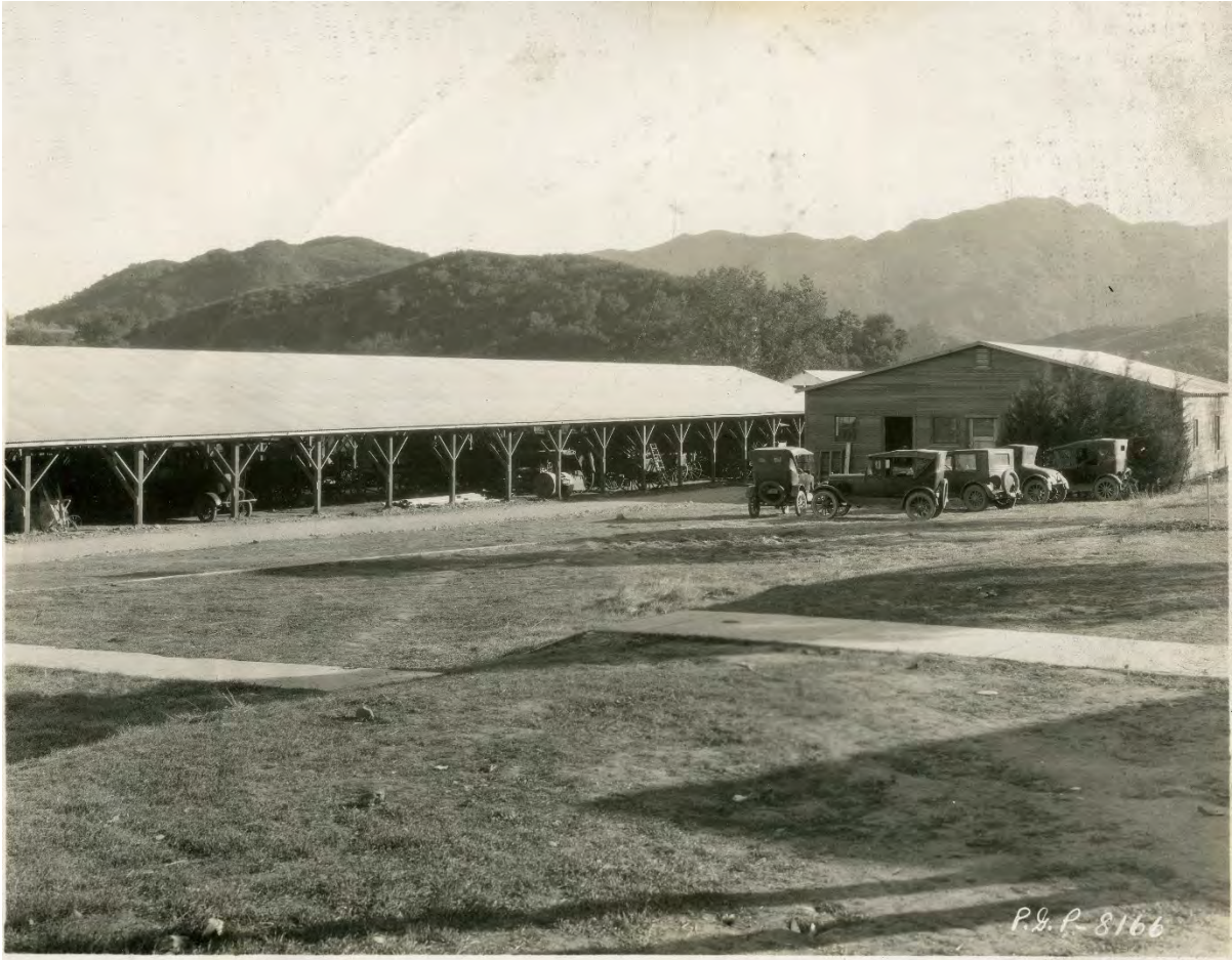
History #2: Prop shed and paint and electrical shop looking south/southeast, circa 1927. (Source: MARC WANAMAKER/BISON ARCHIVES)
