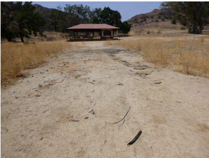
Impacts 2: Debris on Hertz Western Town Road (NPS, August 2021).
