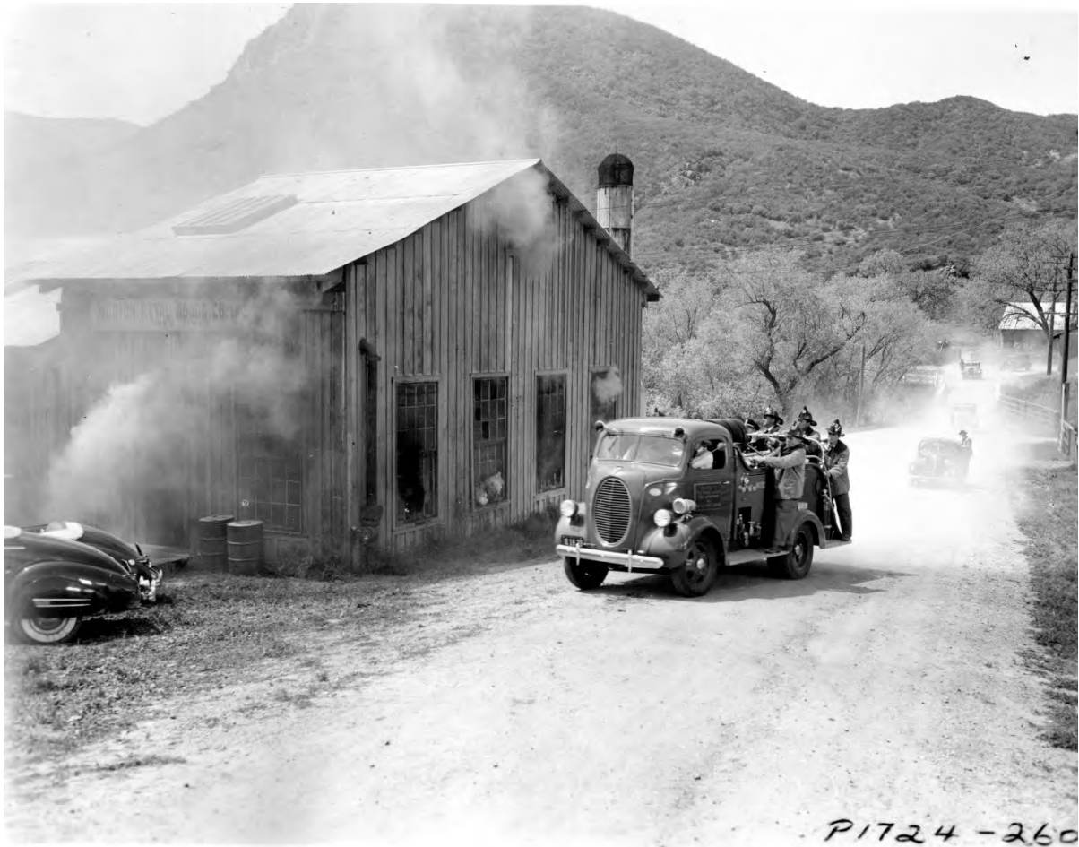
History #3: The Mill/Carpenter Shop during filming in 1941, looking west. The incinerator is visible over the building's roofline. The Medea Creek Bridge and barn are visible in the background along with Sugarloaf Peak. (Source: MARC WANAMAKER/BISON ARCHIVES)
