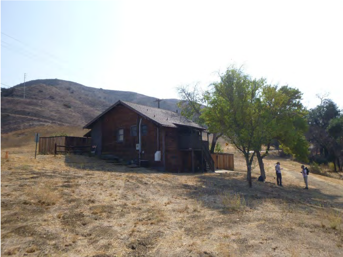
Buildings and Structures 3: Fire Patrol Station House, northwest elevation (NPS, August 2021).
