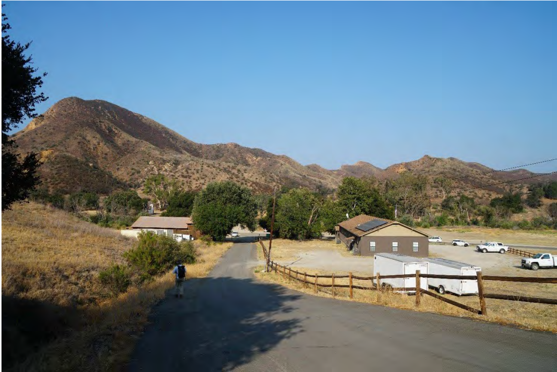
Circulation 1: Original Main Ranch Entrance Road, facing west looking at the Main Ranch Cluster (NPS, August 2021).
