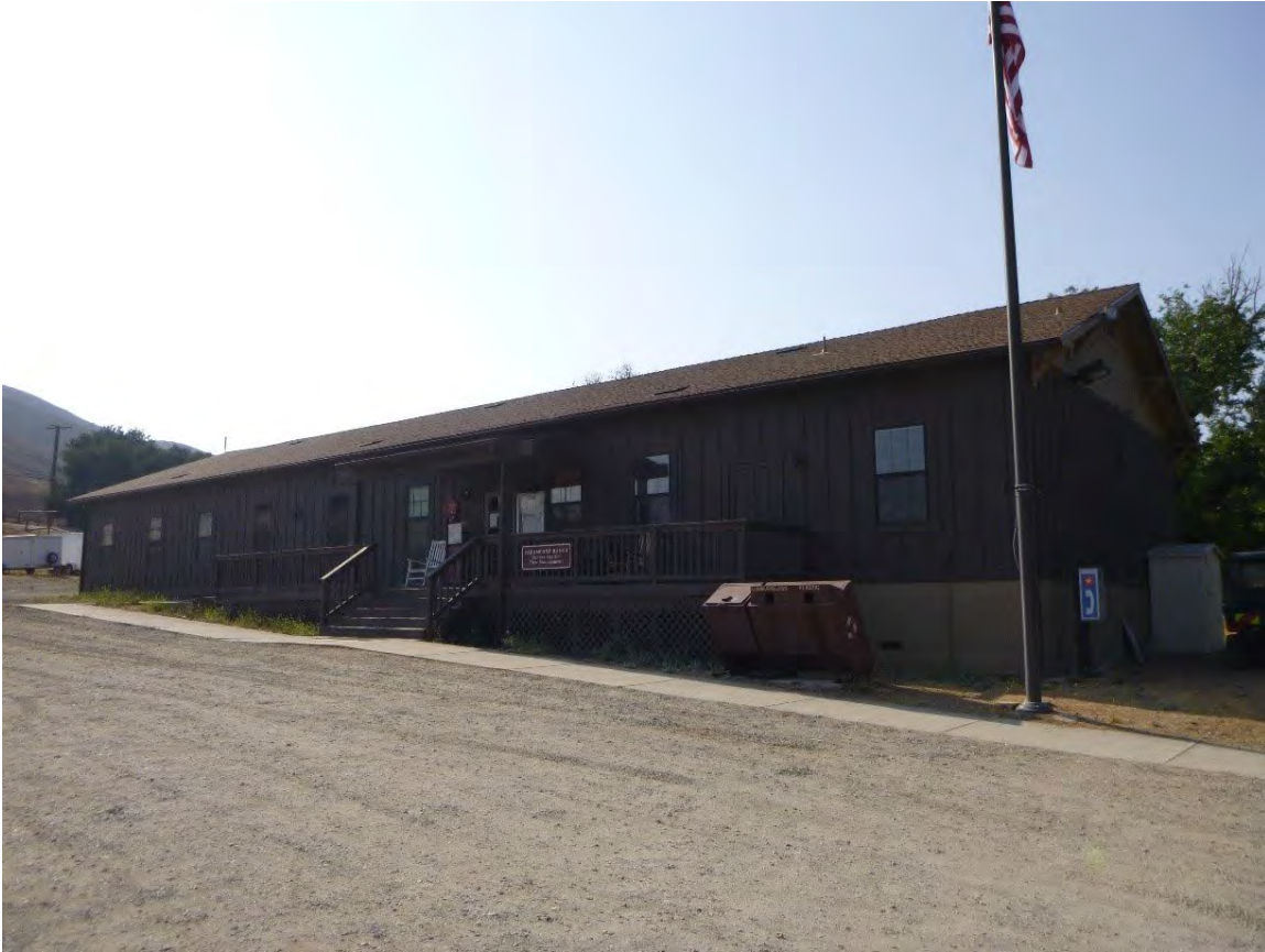
Buildings and Structures 11: Longhorn Building, north elevation (NPS, August 2021).
