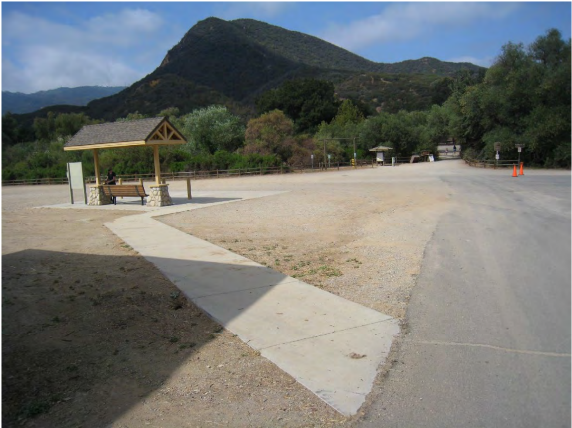
Circulation #5: Concrete sidewalk and pad associated with the shuttle stop (NPS, 2015).
