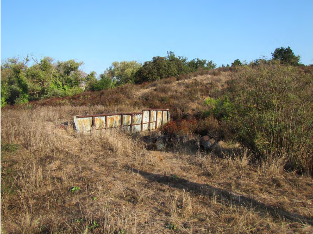
Archeological Sites #3: Photograph looking northwest showing a pipe and sheet metal retaining wall. The construction date and function of the wall is unknown; however, it is located in proximity to the concrete pad noted above (NPS, 2015).
