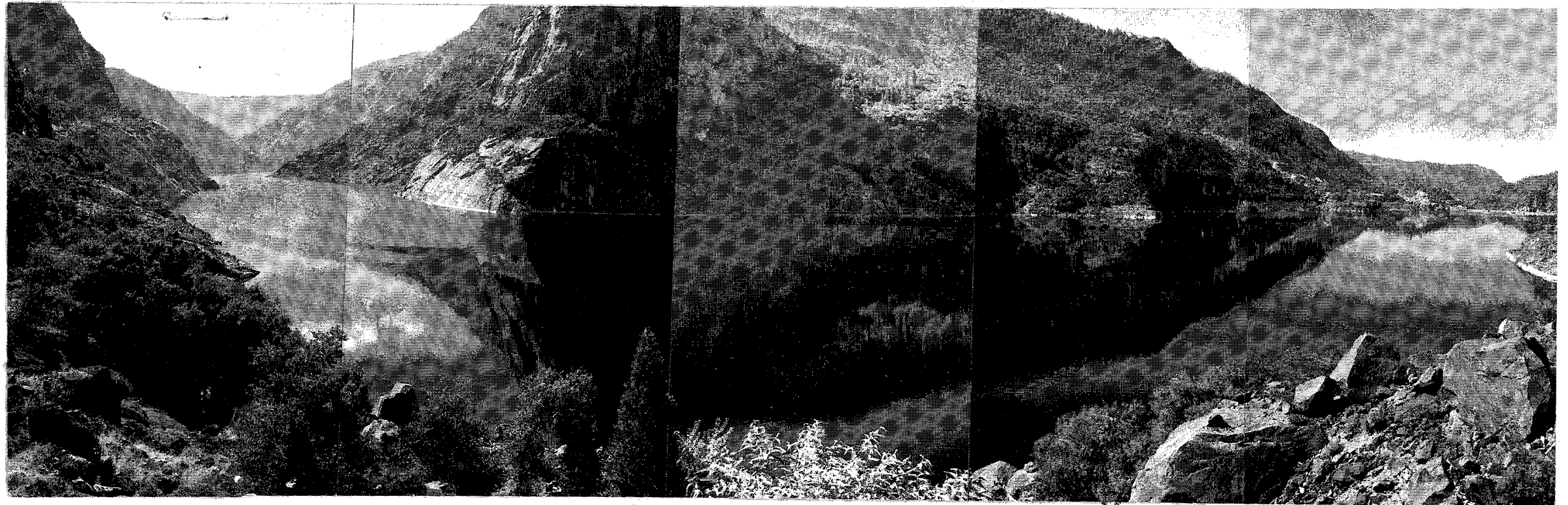
Albani Fig. 45. Hetch Hetchy Reservoir as seen from opposite Kolana Rock. The dotted line indicates a previous water level; when the present construction is completed, the level will be 85 feet higher yet. K- Kolana Rock; D- O'Shaughnessy Dam; E- excavation in side of mountain to obtain rock for cement work.
