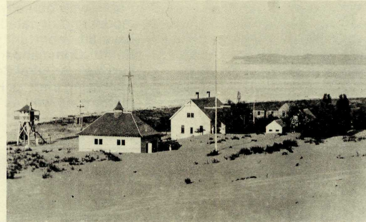
Sleeping Bear Point Life-Saving Station, 1920 — Note drifting sand engulfing buildings.
