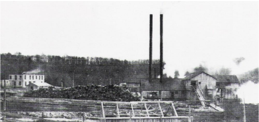
Crescent Hotel/Boarding House and Sawmill ca. 1910
