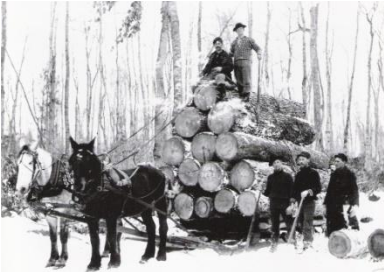
Loading gang and team after loading a sleigh
