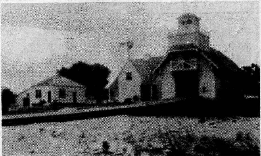
North Manitou Island Life-Saving Station
