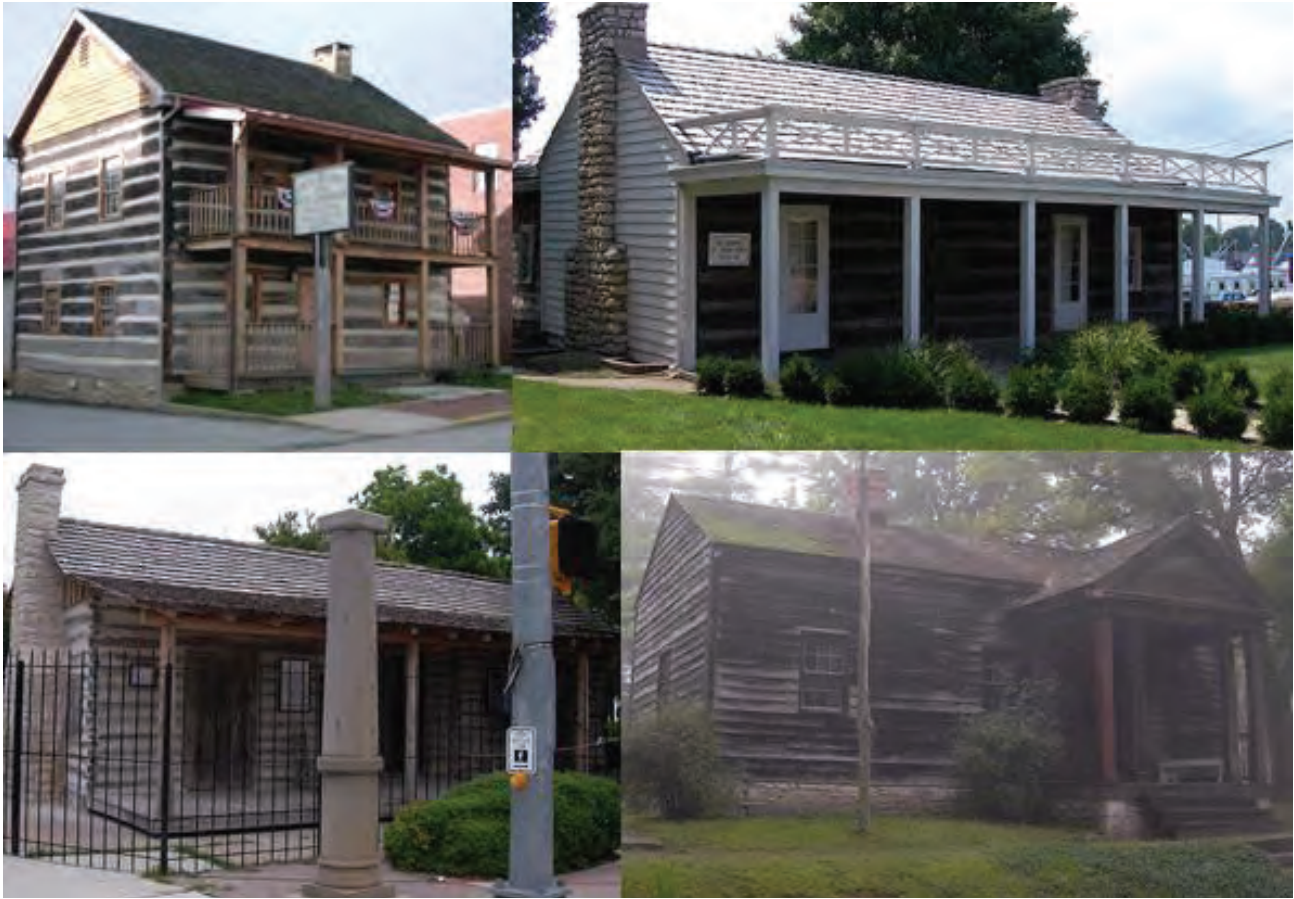
Figure 22 (upper left): Greene County, Pennsylvania Court House (1796); Figure 23 (upper right): Jackson County Courthouse, Independence, Missouri (1828); Figure 24 (lower right): “Old Saline Courthouse” in Arrow Rock, Missouri (ca. 1840); Figure 25 (lower left): Comanche County Courthouse in Comanche, Texas (1856)
