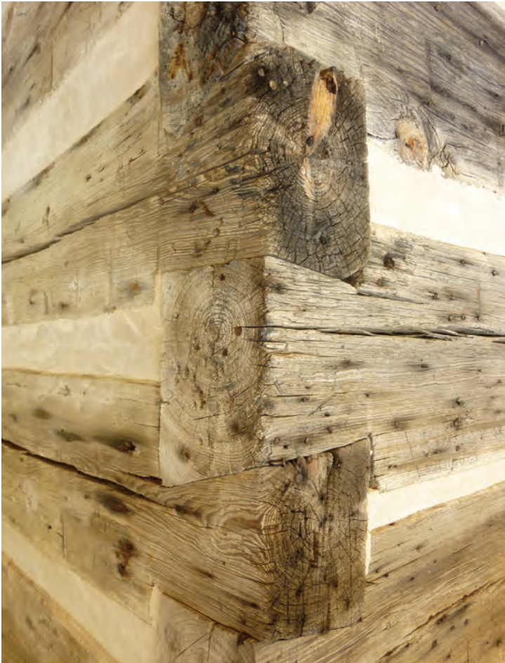
Figure 16: Half-dovetail notch, Wolf House.
