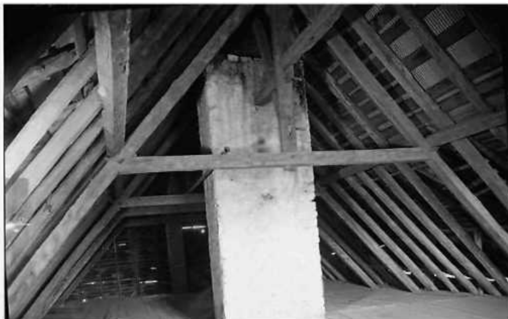
Interior of attic showing Norman trusses. HABS
