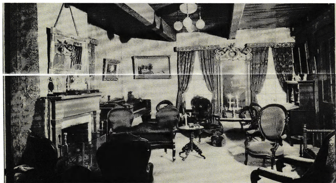
This 1949 photo from the Historic American Buildings Survey (HABS) shows the home fully furnished and decorated in a mid- to late-Victorian style.
