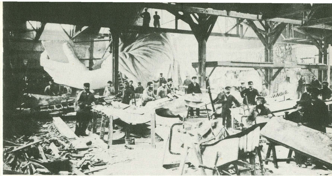
Sheet copper for statue being hammered into shape in Paris workshop
