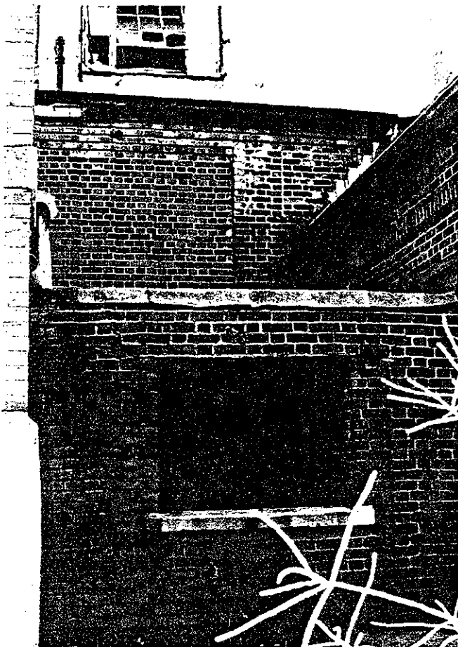
4.12 Kitchen and Laundry Building, Passageways E and F
