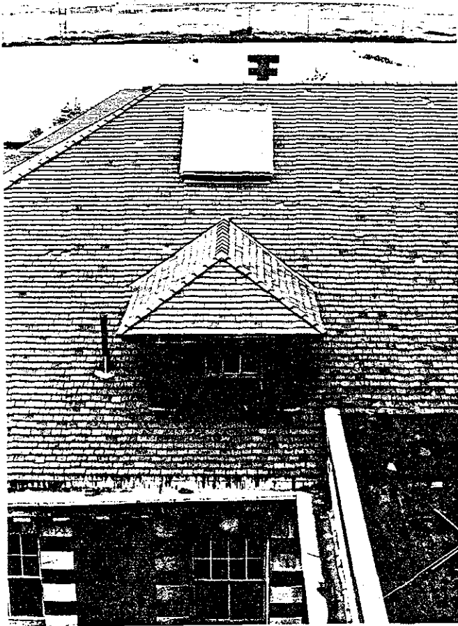
4.5 Kitchen and Laundry Building, Dormer and Skylight Detail
