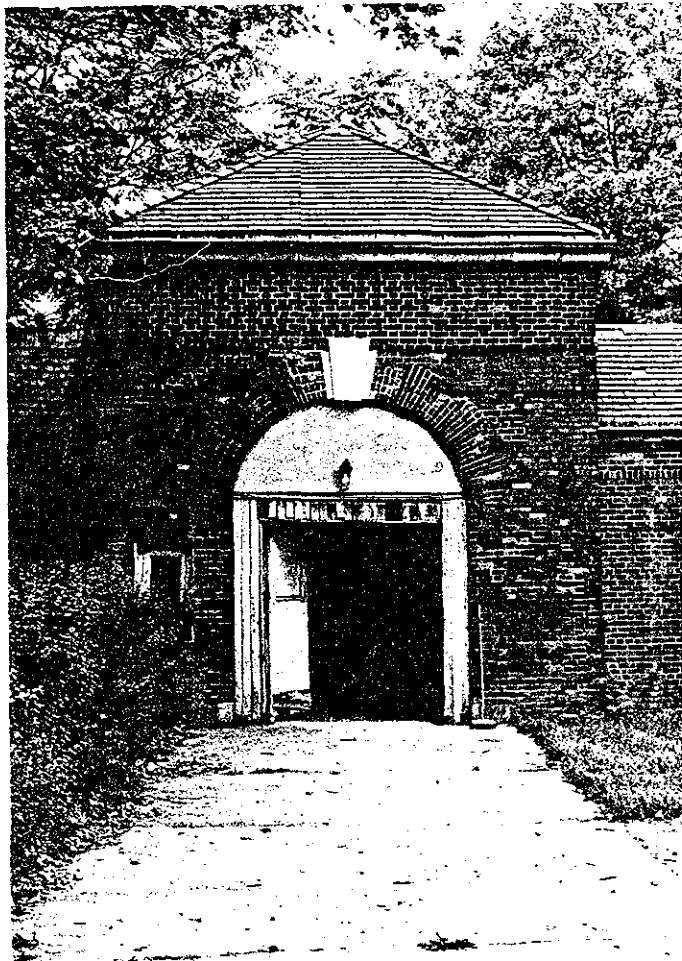
16.2 Passageway, East Elevation of End Pavillion in Part A
