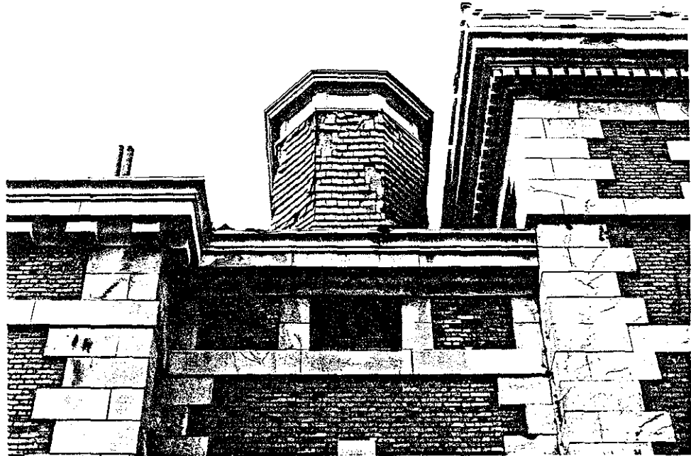
19.2 Hospital #1. Loose and missing tiles on skylights.
