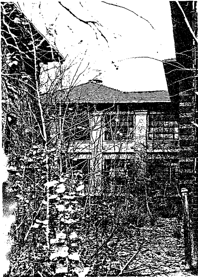
27.2 Passageway, Section D
