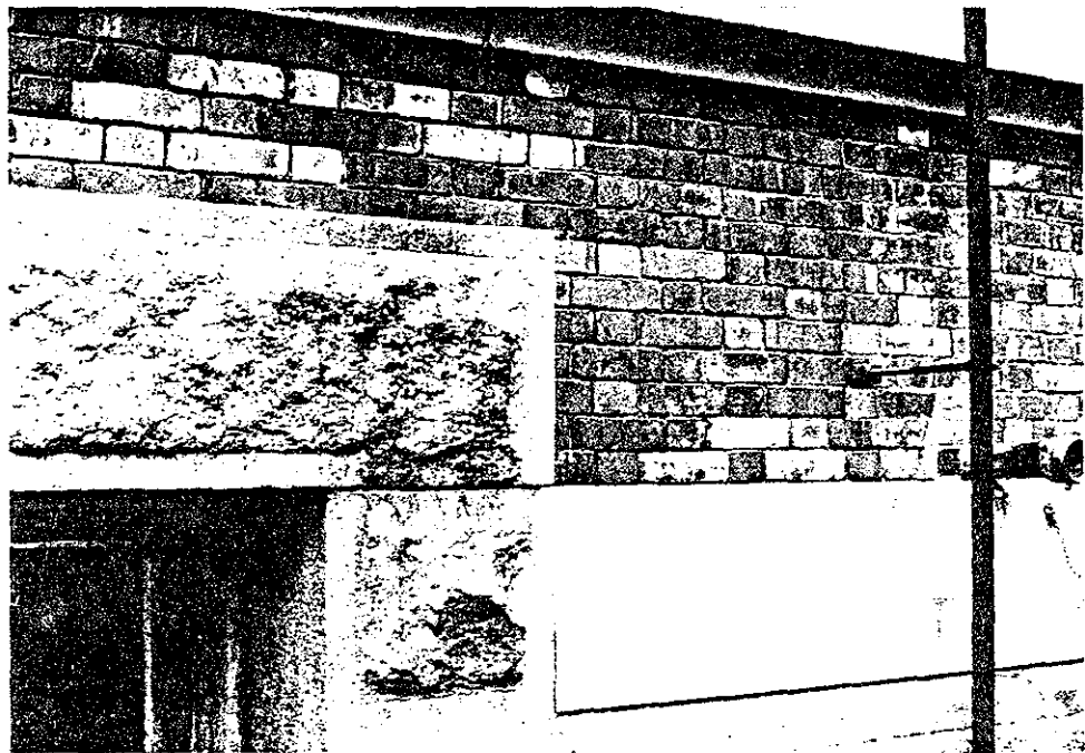
19.3 Hospital #1. Efflorescence and open joints above water table.
