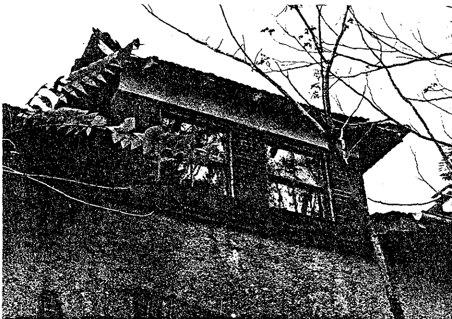
39.2 Wards 29/30. Damaged eaves in north dormer.
