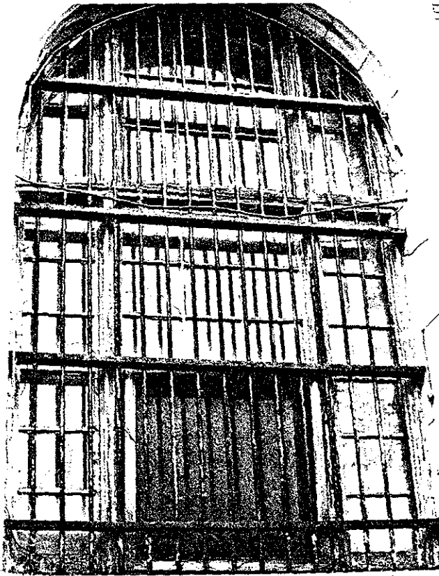
1.14 Main Building, Original Window Grill
