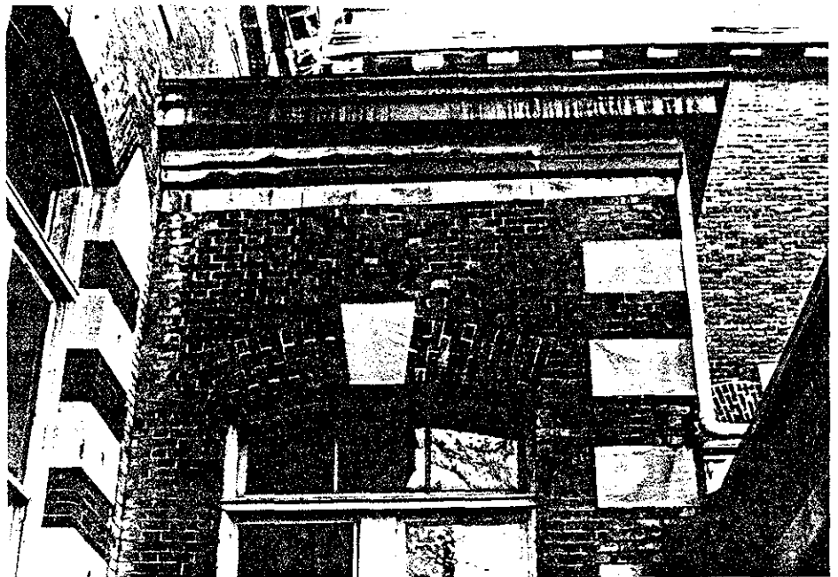
4.4 Kitchen and Laundry Building. Loose and missing brickwork on northwest wall above cellar door resulting from missing drainpipe.
