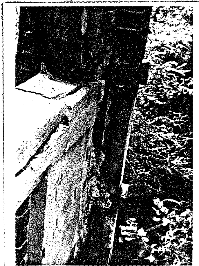
Damaged Column at 2nd Floor Balcony
