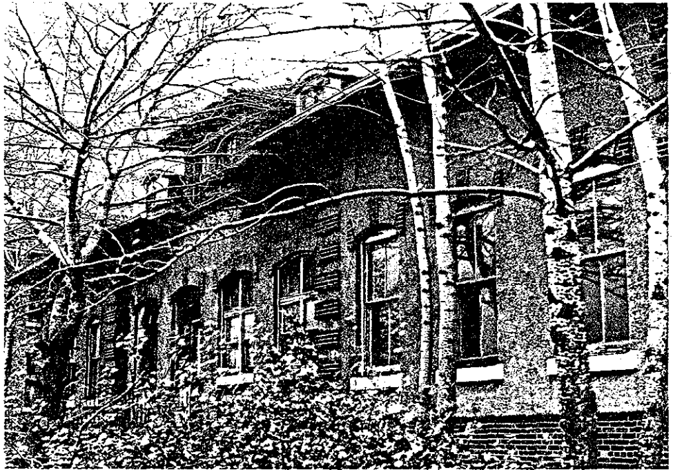
38.1 Wards 27/28, South Elevation
