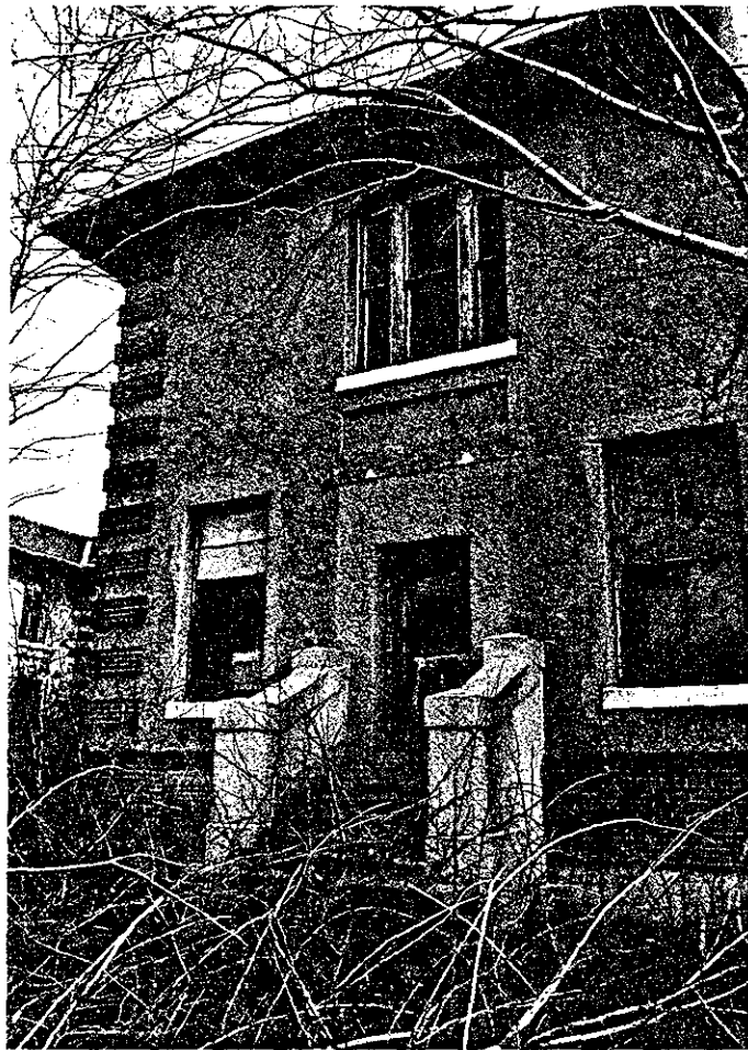
36.3 Wards 23/24, South Elevation
