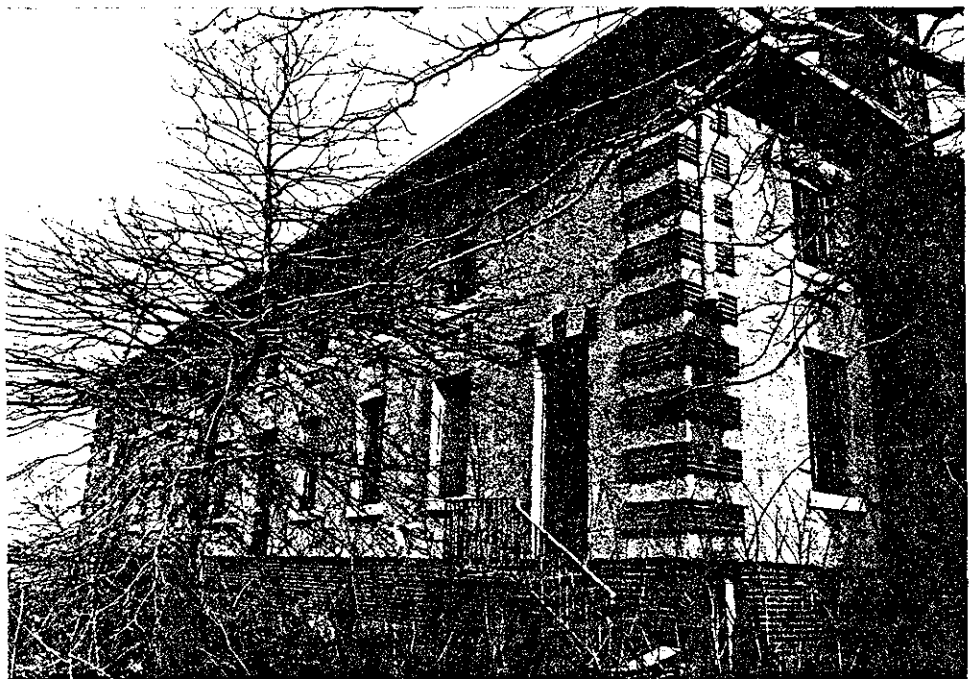
24.2 Powerhouse and Storage, South Elevation From East
