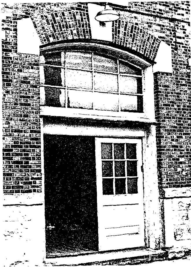
5.3 Powerhouse, West Doorway
