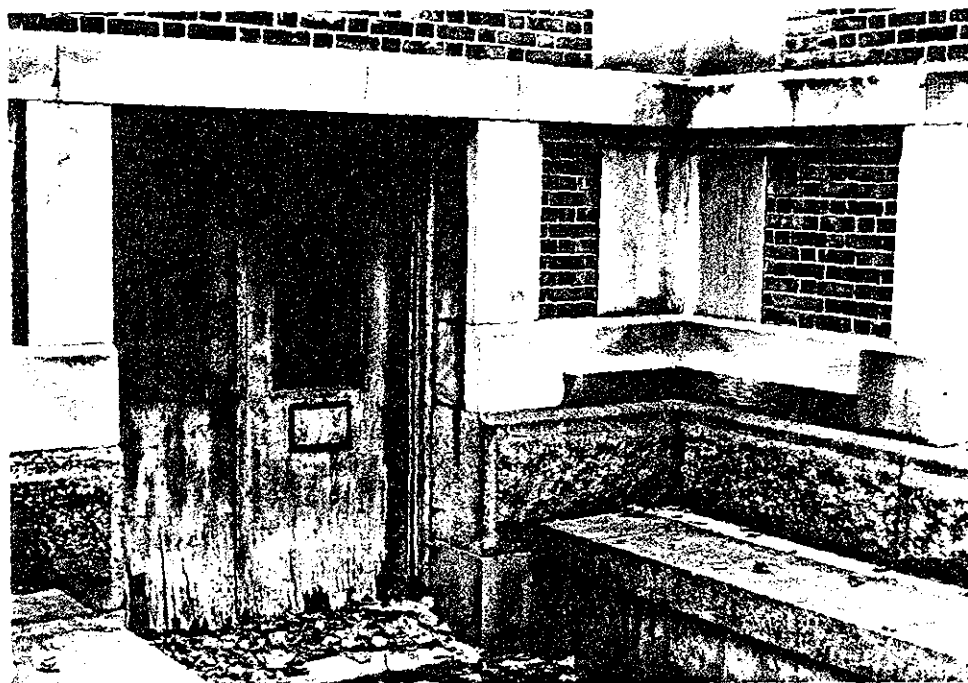
21.3 Hospital #2. Split and warped cellar doors.
