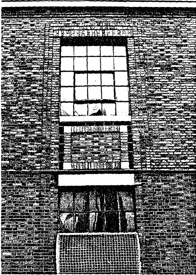
10.2 Bakery and Carpentry Building. Typical window bay showing cracked brickwork around lintels.
