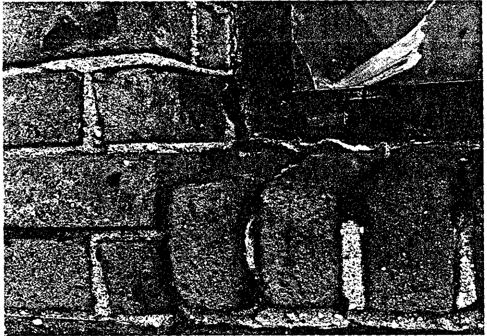
16.8 Passageway. Deteriorated brickwork on west side of section D.
