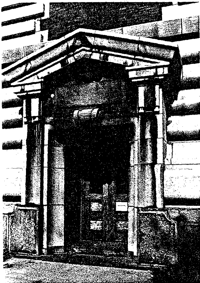
1.7 Main Building, Southwest Tower Door
