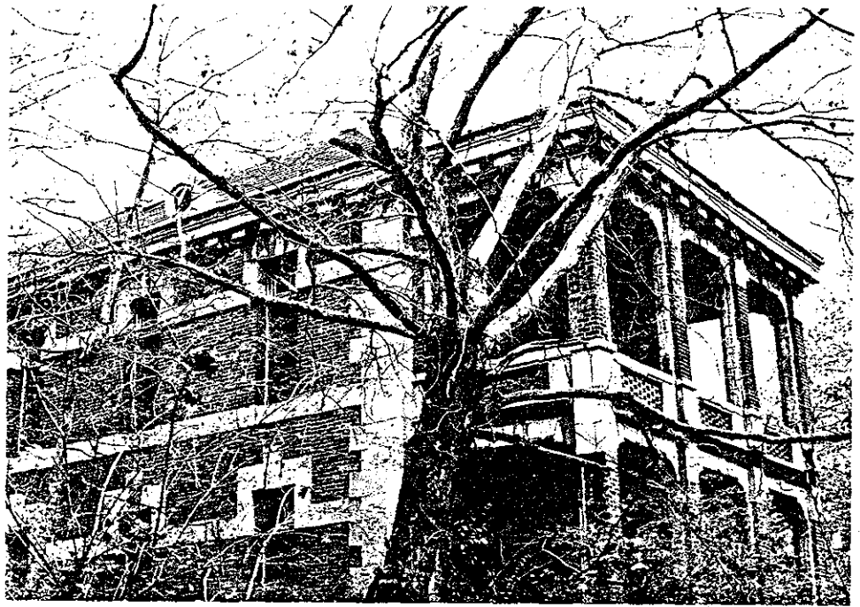
21.4 Hospital #2, Southeast Wing
