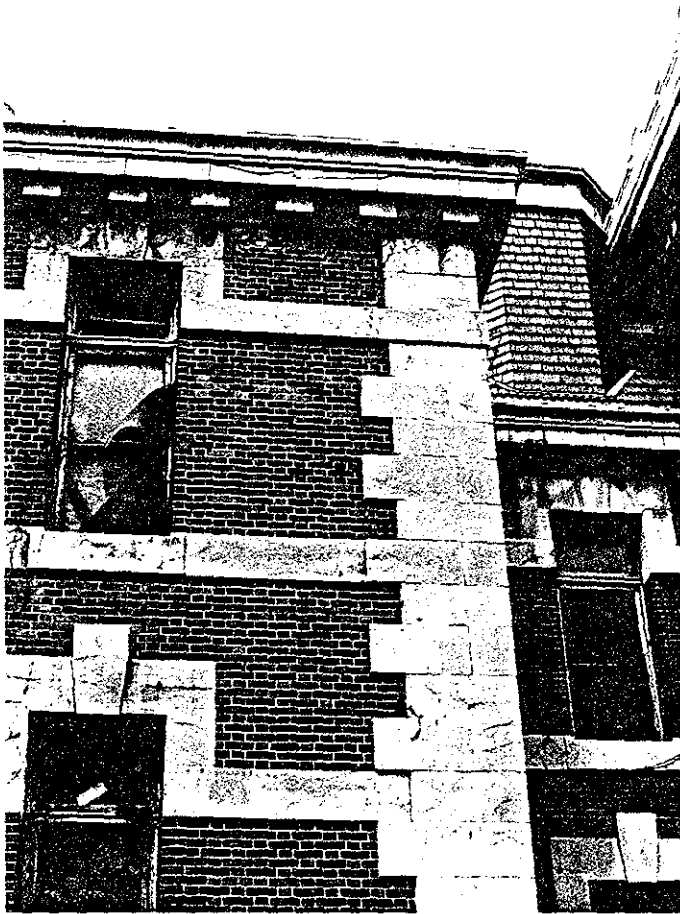
21.1 Hospital #2. Cracked terra cotta cornice blocks.
