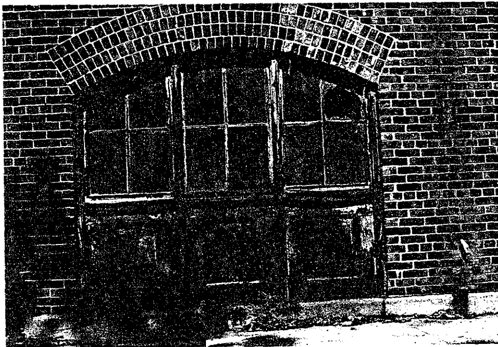
13.1 Passageway. Typical window unit, showing corroded sills and panels. Downspout to the right is missing.
