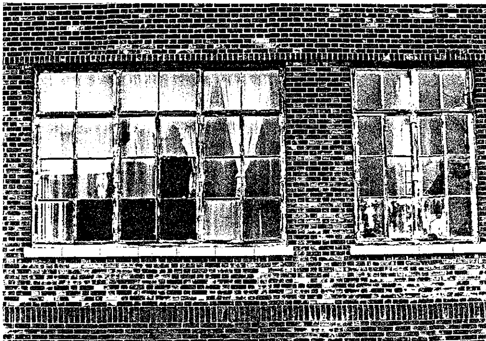
15.3 Immigration Building, Window Units
