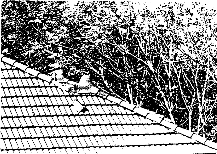
39.1 Wards 29/30. Missing tiles or open joints at ridge cap allow water to flow in along ridge battens.
