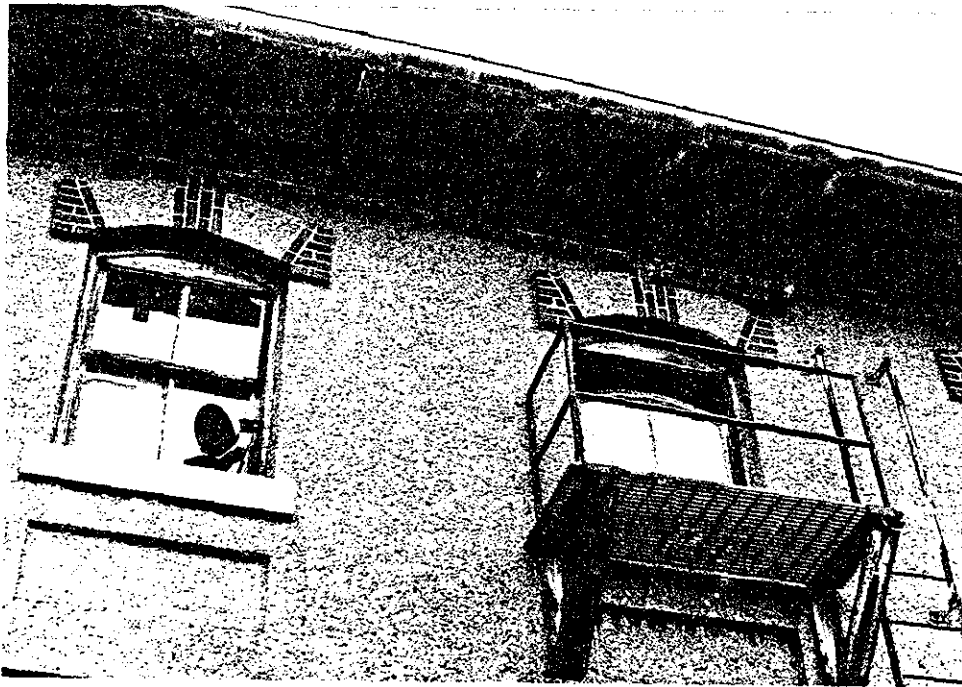
24.3 Powerhouse and Storage, Second Floor Window Detail
