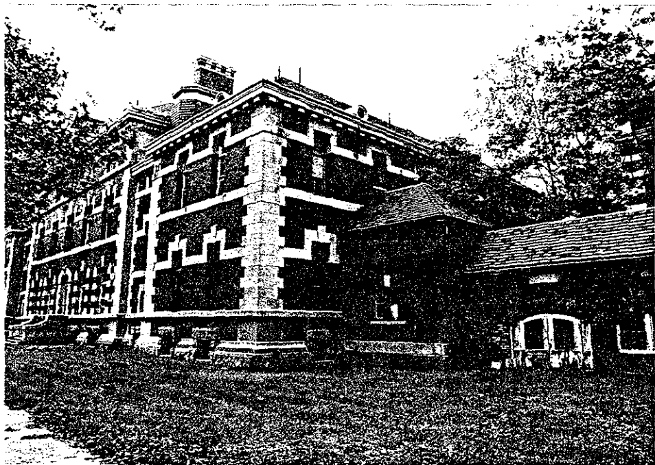
19.2 Hospital #1, Northwest Corner
