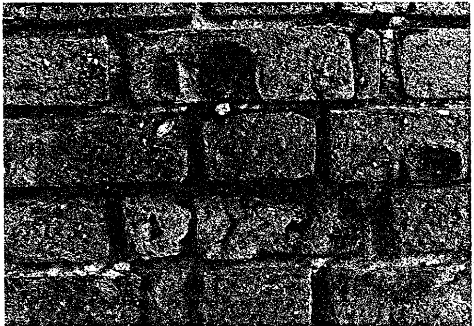
16.9 Passageway. Open joints on west side of section D.
