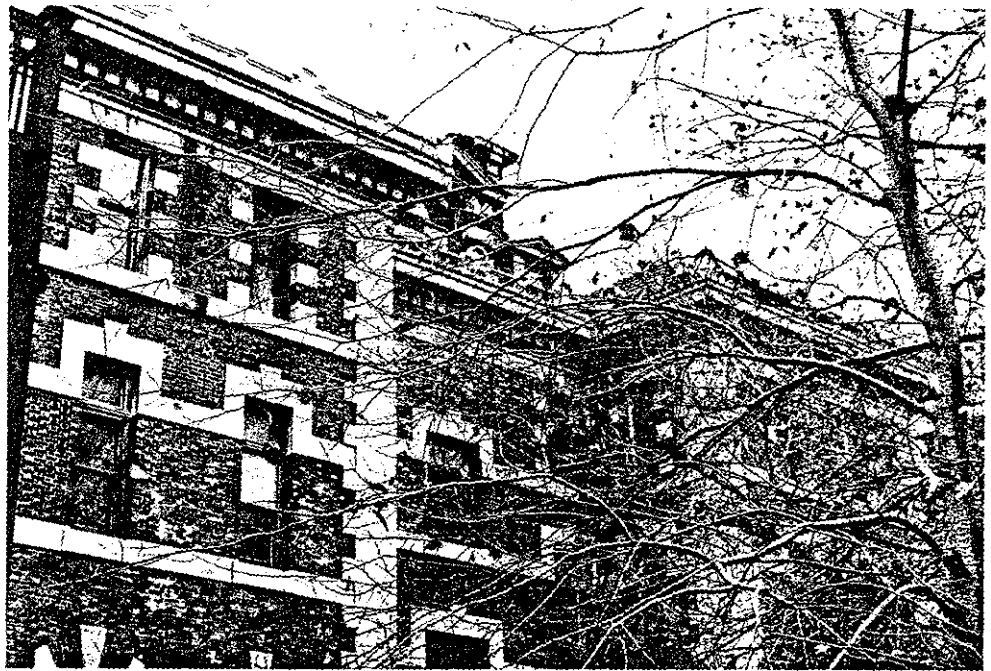
20.3 Administration Building, South Elevation
