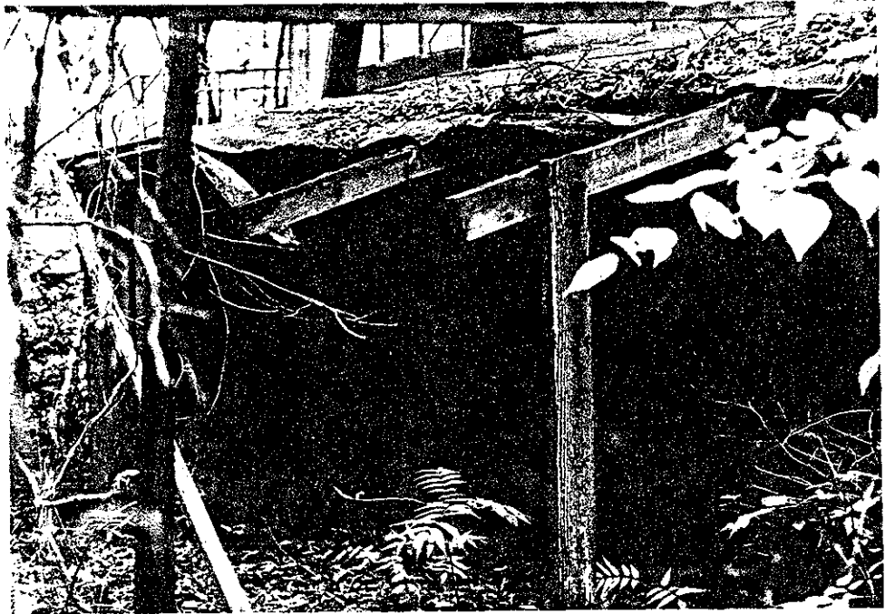
27.6 Passageway. Lean-to on west side of Section E.
