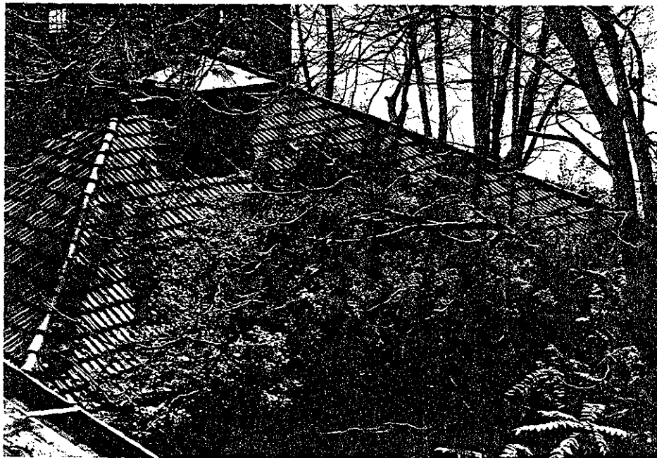
33.1 Kitchen. Roof covered with vegetation.
