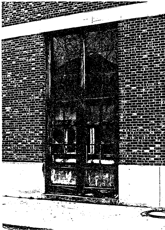
14.4 Ferry Building, South Elevation Door
