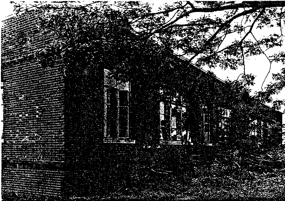
15.2 Immigration Building, Northeast Corner
