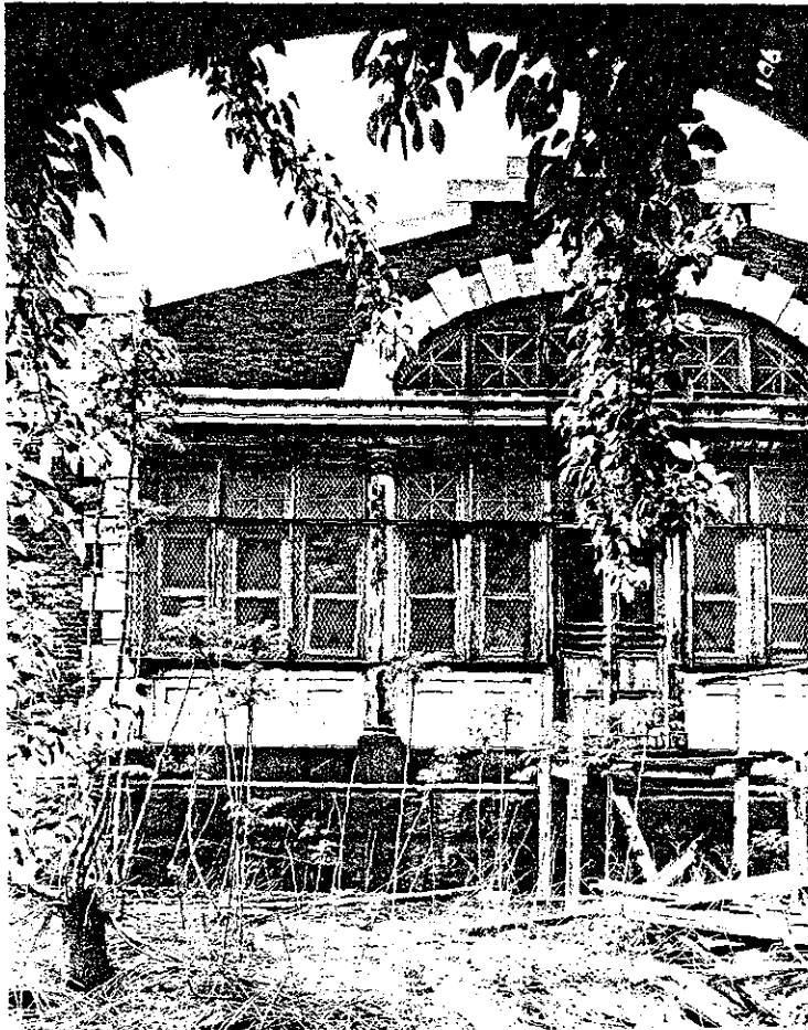
1.12 Main Building, Central Bays of North Elevation on Ticket Office
