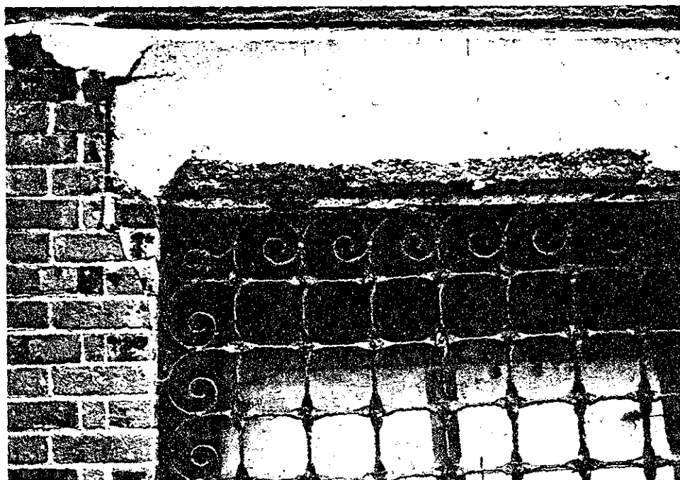
21.4 Hospital #2. Corroded ironwork and lintels on south porches.
