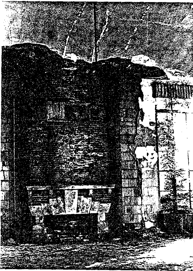
22.3 Recreation Hall. Damage to interior finishes around central chimney.
