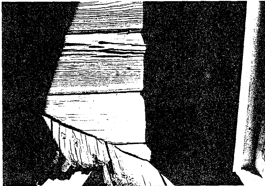
41.1 Staff Headquarters. Split and checked wood dormer sheathing. Caused by exposure through open windows, this condition is similar to that found in Buildings #26 and #32.
