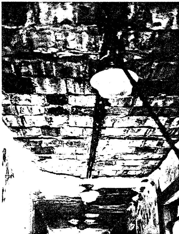
Structural clay tile fireproofing.
