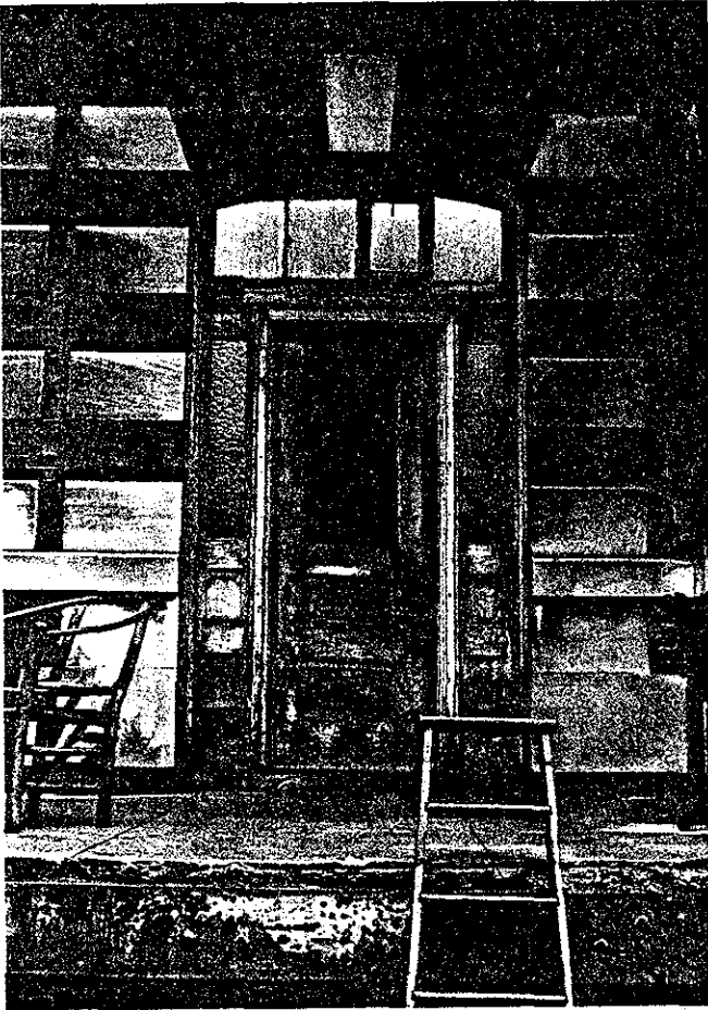
4.3 Kitchen and Laundry Building, Door Opening Onto South Porch
