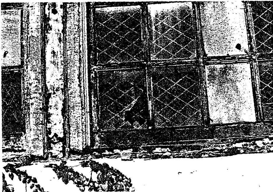
3.2 Baggage and Dormitory Building, North Wing. Corrosion of window sill and muntins.
