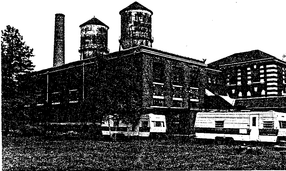
10.2 Bakery and Carpentry Building, Southwest Corner
