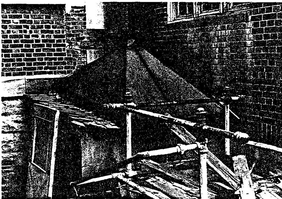
4.8 Kitchen and Laundry Building, Shed Beside Northwest Cellar Entrance
