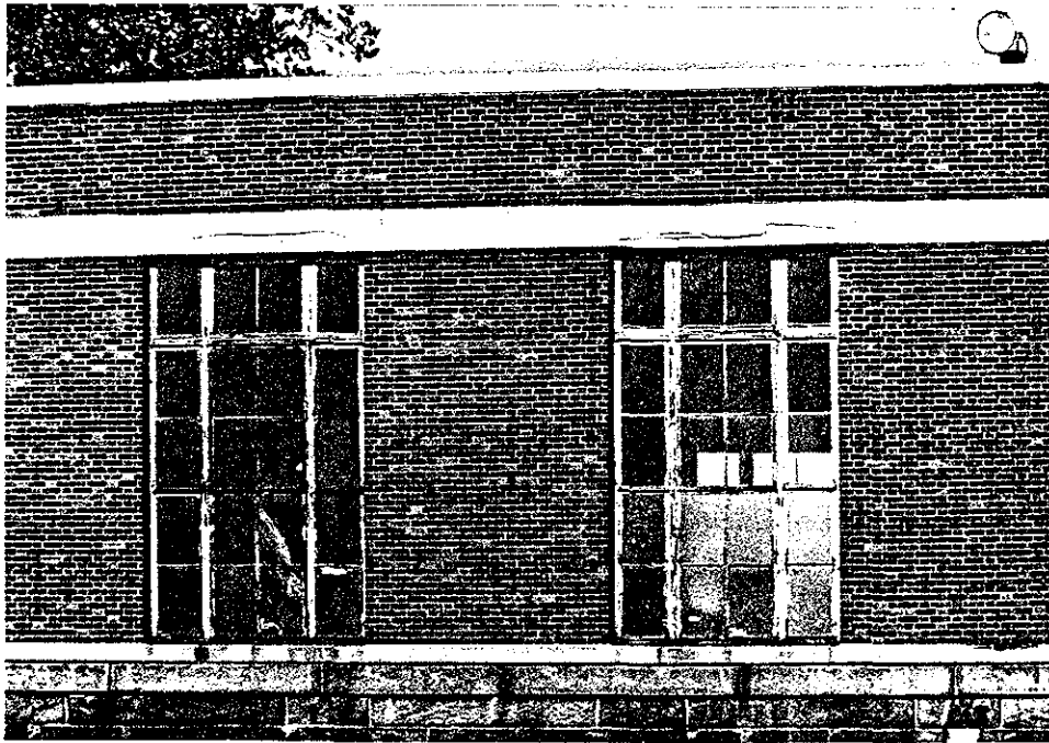
14.3 Ferry Building, East Elevation Window Units
