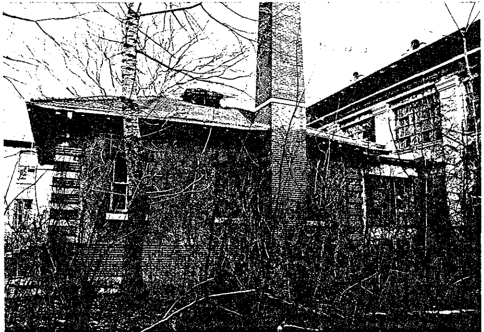
33.3 Kitchen, East Elevation.
