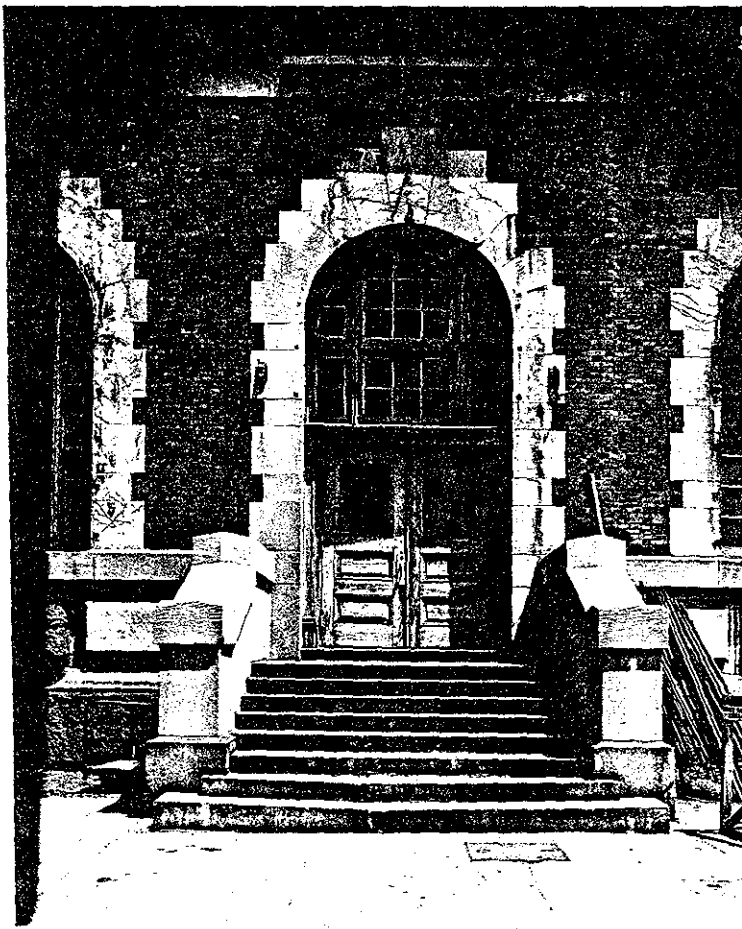
1.5 Main Building, South Entrance
