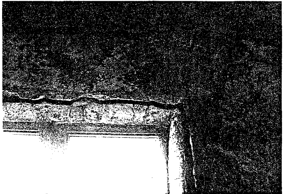
4.6 Kitchen and Laundry Building. Lintel condition on interior of Passageway D.
