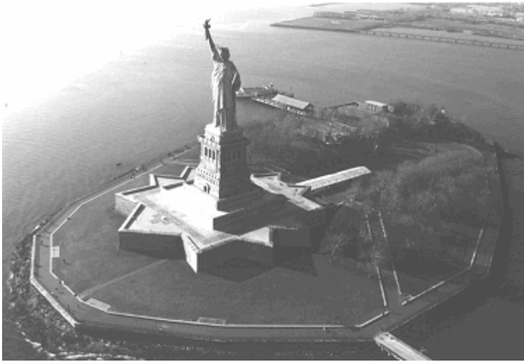
Liberty Island c.2000. Although Liberty Island underwent restoration in 1986, the original fabric of the plantings, circulation system, spatial organization, view sequence has been retained.
