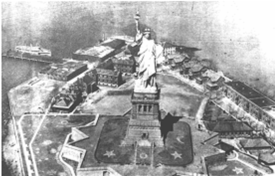
Bedloe's Island during the War Department's tenure in 1933. Later in the year the statue was transferred to the NPS.
