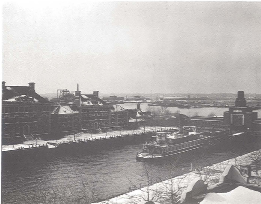
Ferry slip on Ellis Island and New Jersey waterfront in distance.
