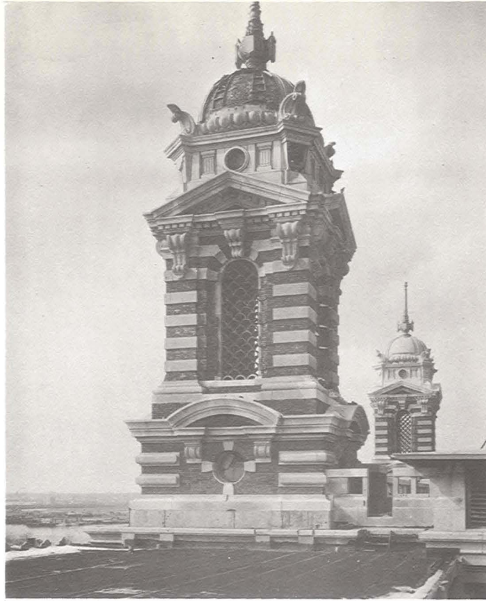
Detail of Tower on Main Building.
